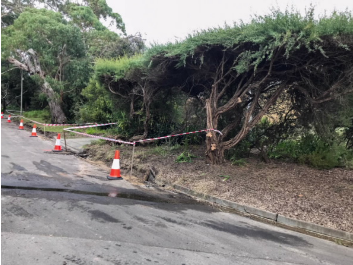
View in 5 May 2023. Shows hump across road to divert water. Note the cracked kerb.
