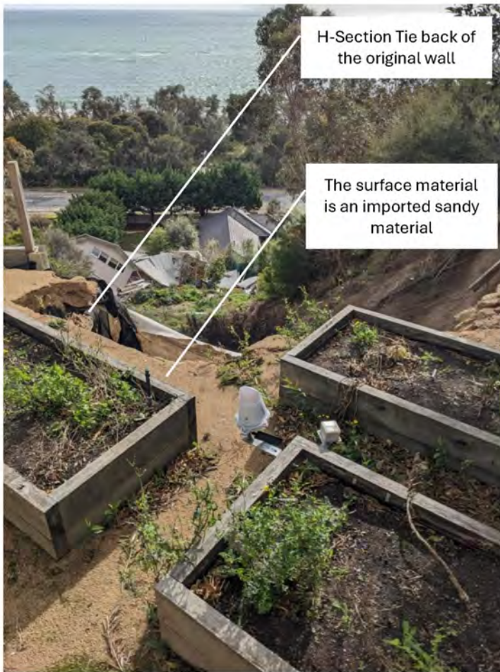
Figure 9: 17/6/25 Photo 06 Looking north from behind the raised vegetable patch, towards the toe debris of the landslide. The tie back of the original retaining wall is visible, as is the white geofabric of the drainage measures of the 'aesthetic' wall
