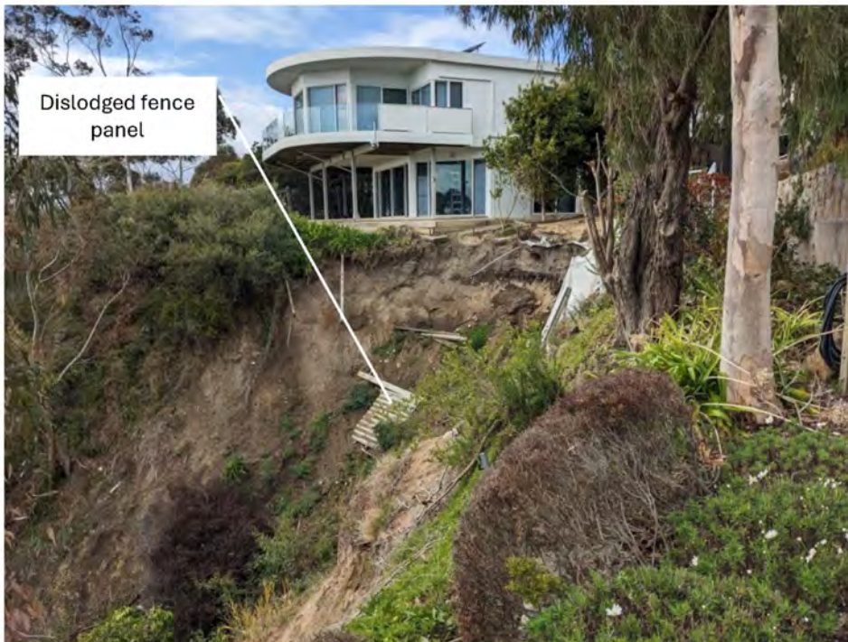
Figure 6: 17/6/25 Photo 03 Looking east showing the upper slope of the escarpment, and assumed extent of slip, showing debris downslope of the backscarp
