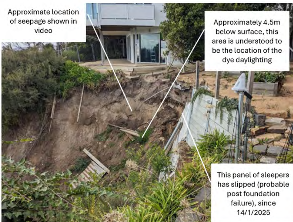
Figure 12: 17/6/25 Photo 09 Looking east showing the location of the seepage videoed by the landowners on 14 January 2025, and location of the dye that was seen daylighting through the backscarp after dye was poured into NDT01/02.
