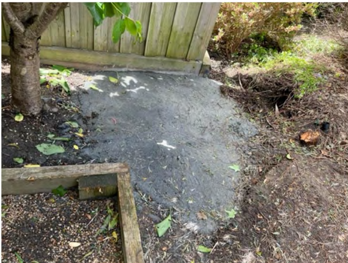
Figure 25: Photograph from email of 22 November 2022, showing detail of sinkhole repair within private land.
