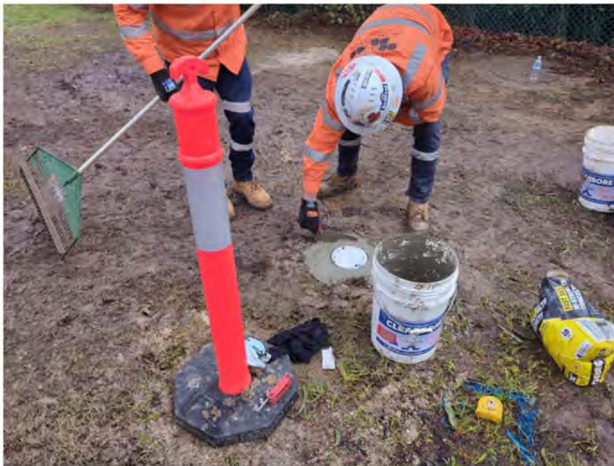
Figure 4: Well installation at BH01
