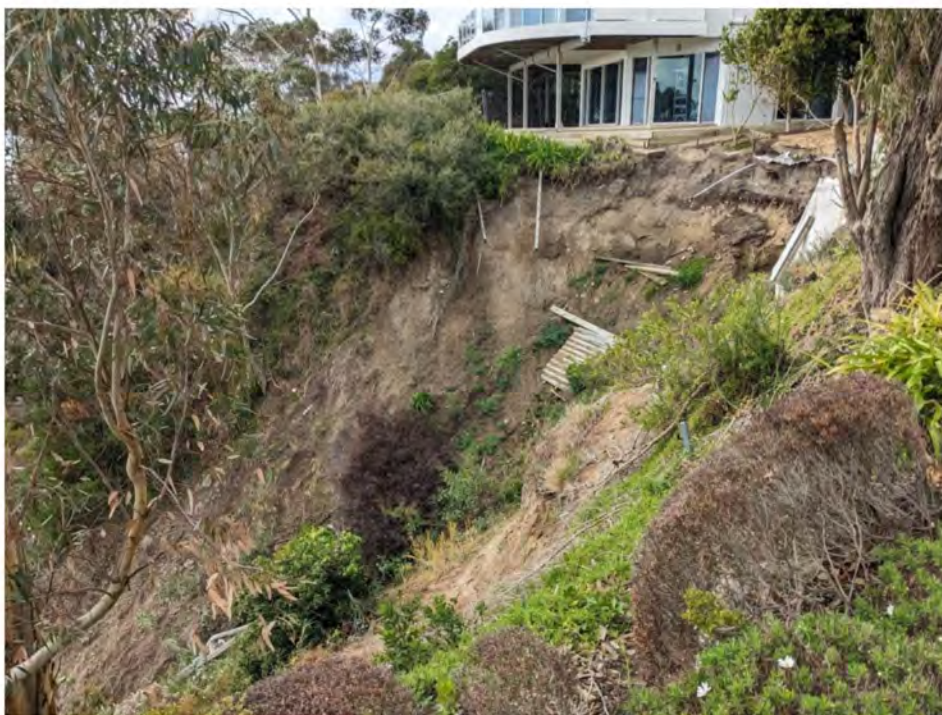
Figure 8: 17/6/25 Photo 04 Looking east showing the detail of the backscarp. Note the vertical nature of the backscarp, approximately 4.5m high
