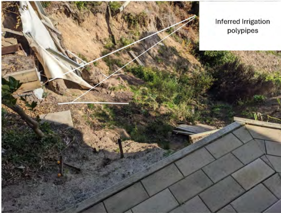
Figure 23: 20/6/25 Looking north west down the failure, showing depth of slope movement.
