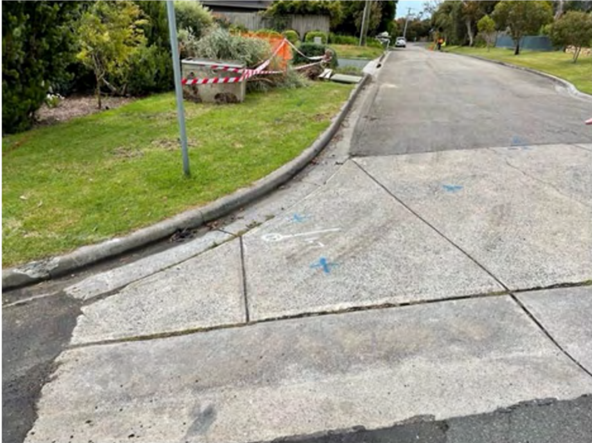
Figure 24: Photograph from email of 22 November 2022, looking north from Coburn Avenue towards Prospect Hill Road showing undulating concrete pavement construction.
