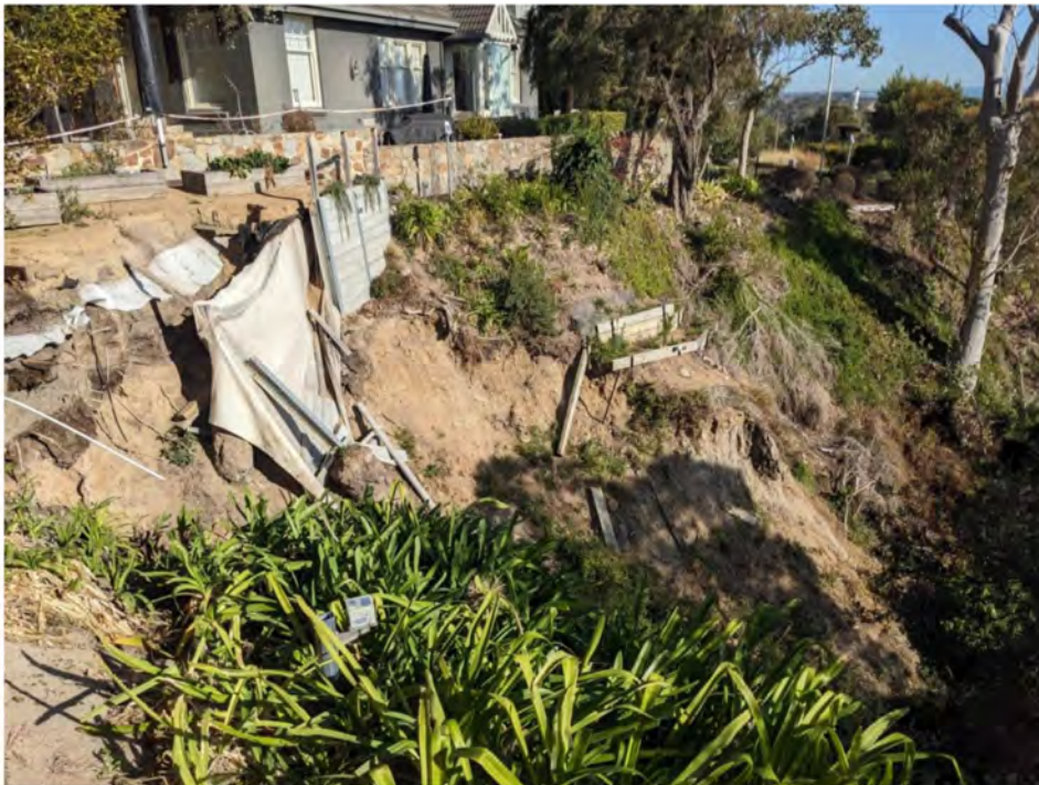
Figure 26: 20/6/25 Looking west from 6 View Point Road. Note the change in geology below the wooden sleepers.
