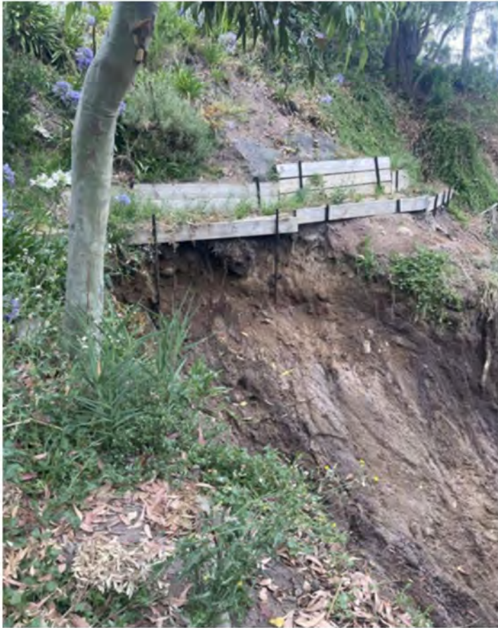
Figure 4: Photo taken by SEW personnel on 6 January 2025 showing detail of backscarp of landslide
