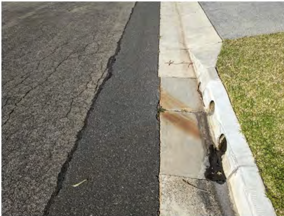
Figure 31: 20/6/25 5 Prospect Hill Road, looking south showing detail of staining flowing from the joint between asphalt and kerb
