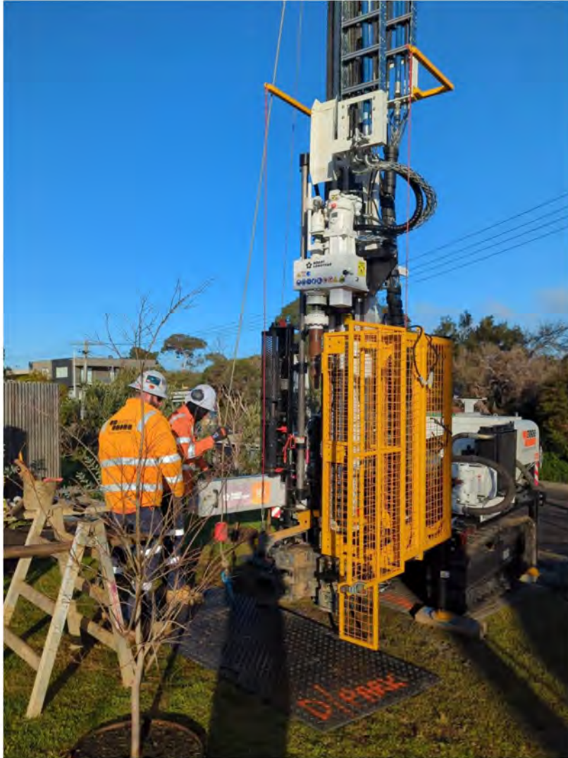
Figure 1: Boart Longyear LX6 drill rig setup
