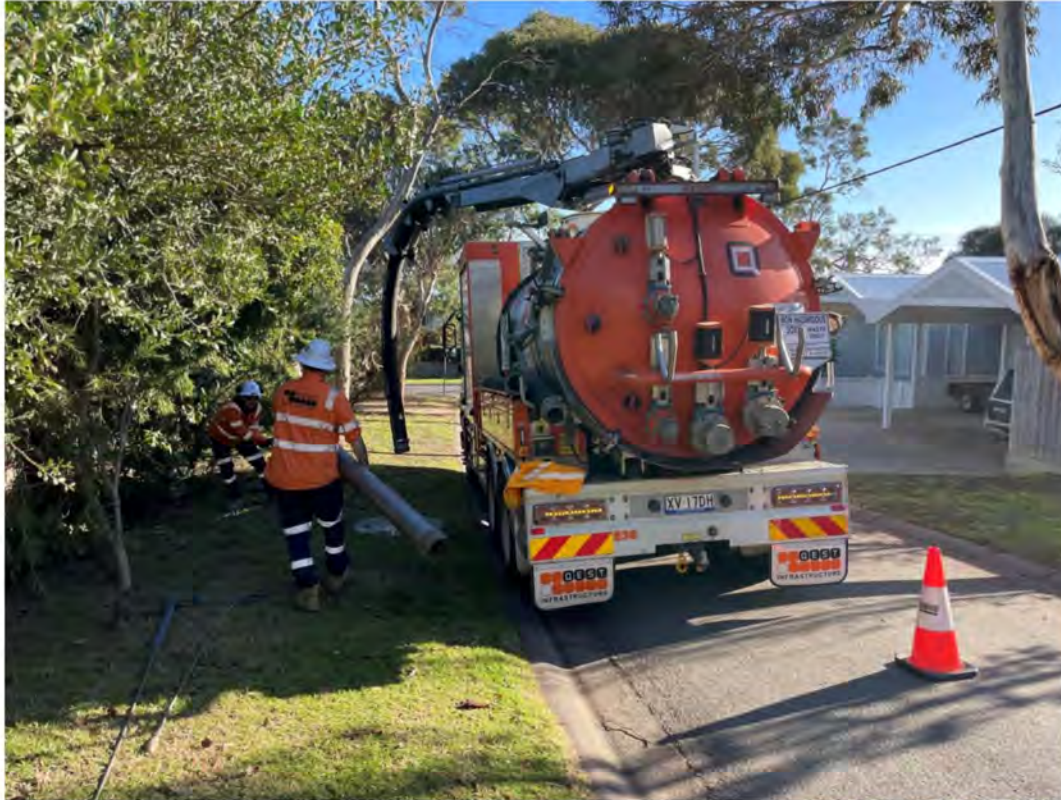
Figure 3: Non-Destructive Digging vacuum truck
