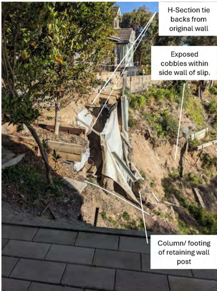
Figure 18: 20/6/25 6 View Point Road looking west along line of retaining walls, showing tie backs, and several irrigation pipes
