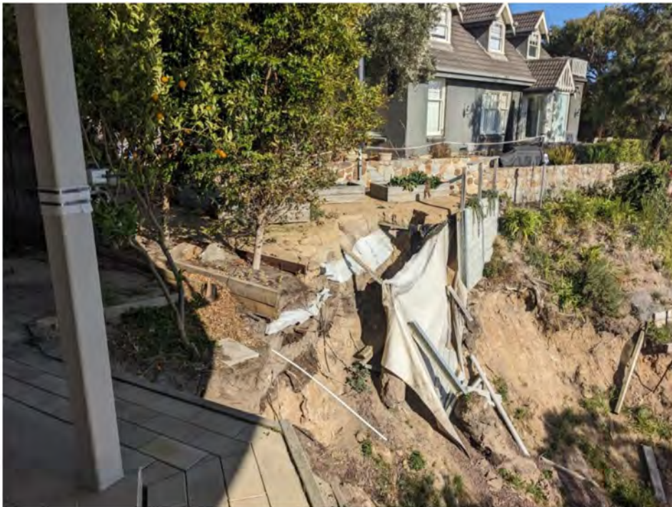
Figure 28: 20/6/25 6 View Point Road looking west. Note the leaning back of the retaining wall posts
