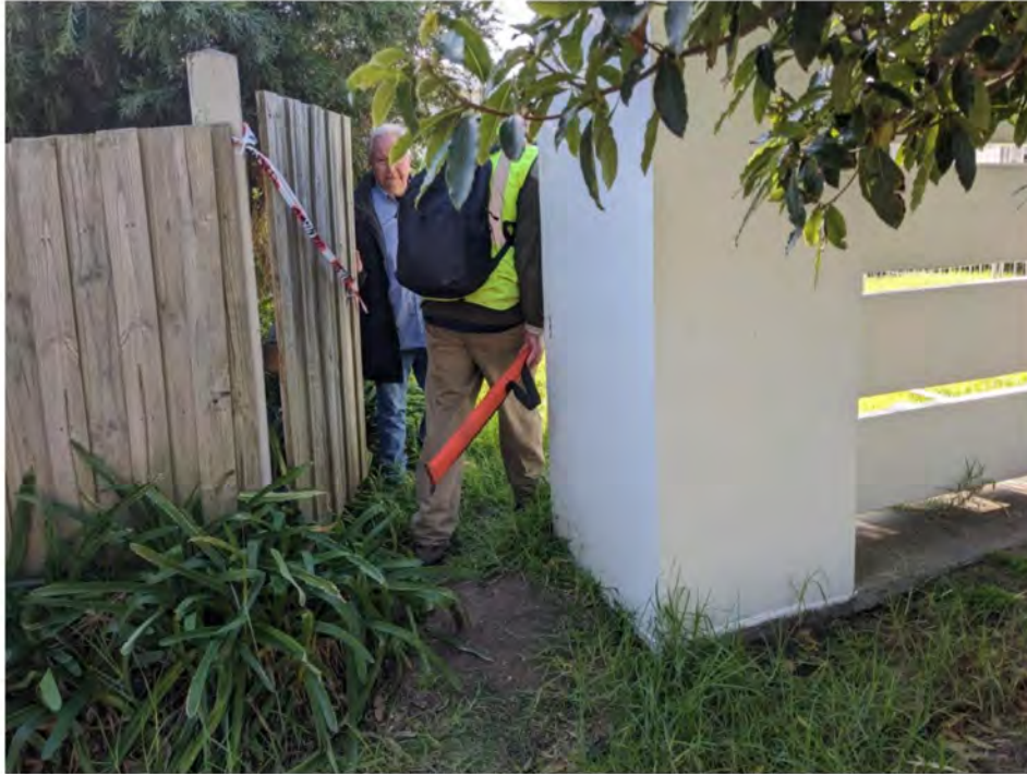
Figure 29: 20/6/25 6 View Point Road looking north showing front gate which has had to be shaved due to toppling concrete pillar.
