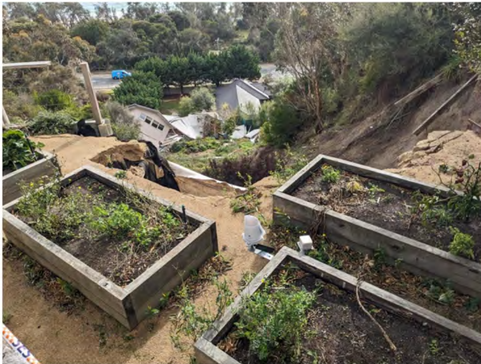
Figure 11: 17/6/25 Photo 08 Looking north over the vegetable garden, showing the crest of the backscarp
