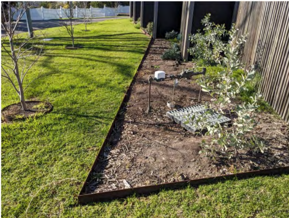
Figure 34: 20/6/25 7 Prospect Hill Road looking east showing gully pot where AG pipes from the property meet, flowing to Stormwater Pit outside No. 11.
