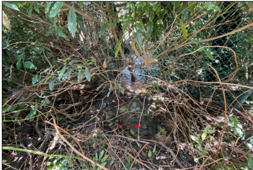
Figure 14 Site photo of burst flow zone, indicating development of a water spout and flow channel at the ground surface of approximately 300mm in diameter (photo date 20/12/2024).
