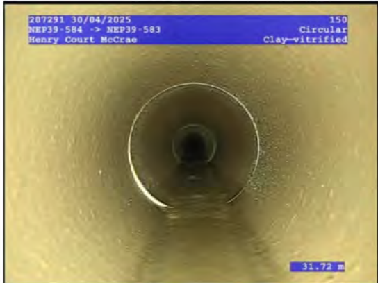
9, 00:15:32, 31.72 Water flow at constant depth, turbid or discoloured water, <5%
