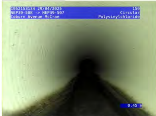
1, 00:00:30, 0.45 Water flow at constant depth, turbid or discoloured water, <5%
