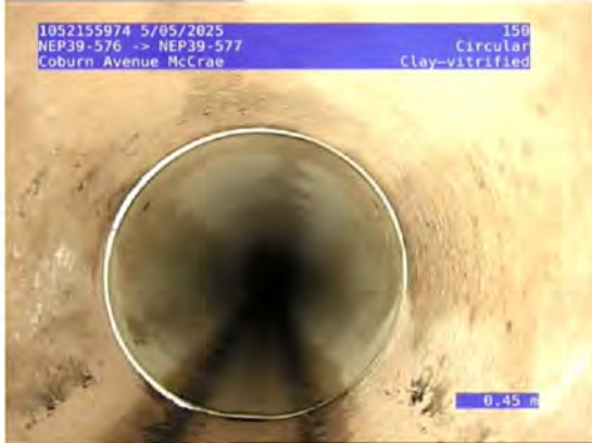
1, 00:00:24, 0.45 Water flow at constant depth, turbid or discoloured water, <5%
