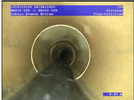
1, 00:00:22, 0.45 Water flow at constant depth, turbid or discoloured water, 5-10%
