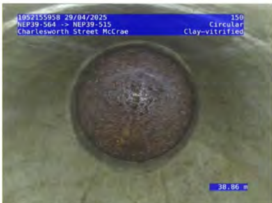
7, 00:14:50, 38.86 Finish node, maintenance hole, Nodename:, NEP39-515
