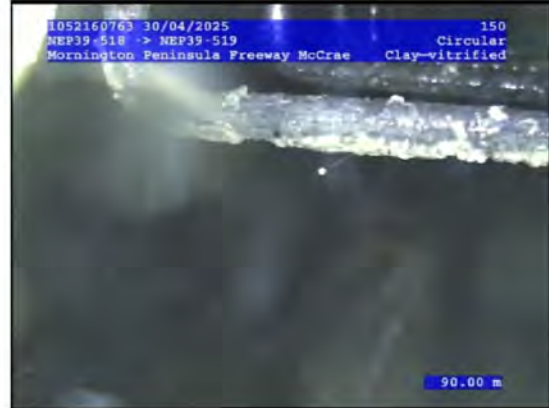
10, 00:46:13, 90.00 Finish node, maintenance hole, Nodename:, NEP39-519
