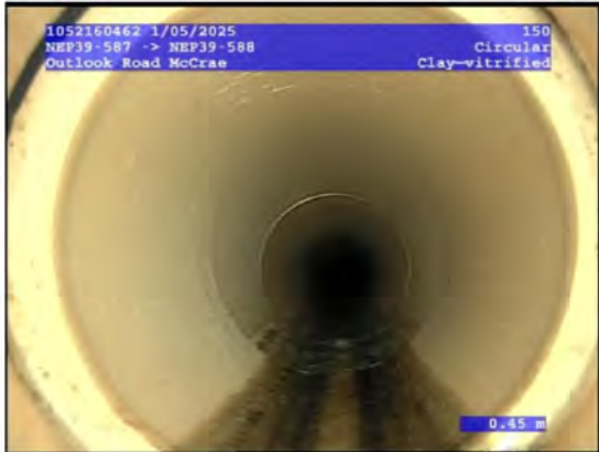
1, 00:00:23, 0.45 Water flow at constant depth, turbid or discoloured water, <5%
