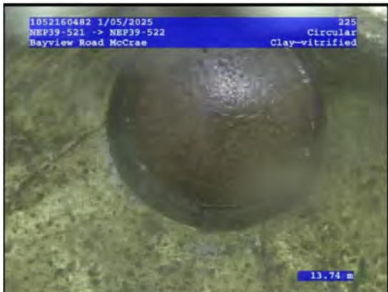
7, 00:06:27, 13.74 Finish node, maintenance hole, Nodename:, NEP39-522
