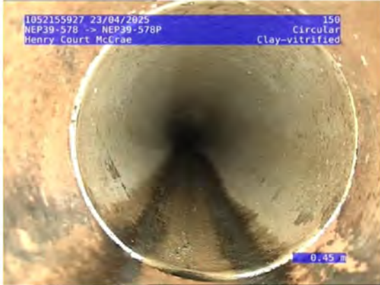
1, 00:00:42, 0.45 Water flow at constant depth, turbid or discoloured water, <5%
