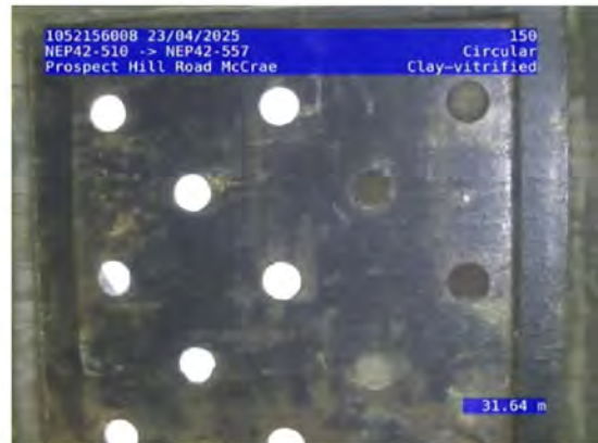
4, 00:10:23, 31.64 Finish node, maintenance hole, Nodename:, NEP42-557
