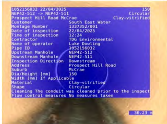
1, 00:00:00, 0.00 Start node, maintenance hole, Nodename:, NEP42-512
