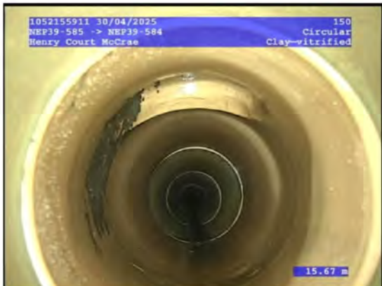
3, 00:06:57, 15.67 Junction, unlined, open, Height/Diameter (mm): 100 at 12 o'clock
