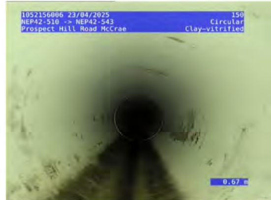
2, 00:00:58, 0.67 Change of conduit material. New material, Polyvinyl chloride
