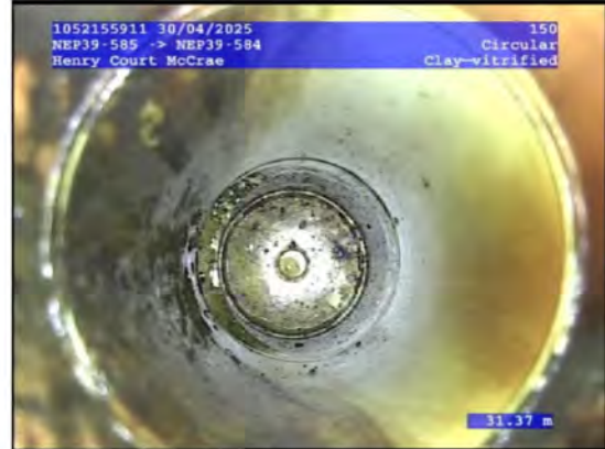
14, 00:15:38, 31.37 Junction, unlined, open, Height/Diameter (mm): 100 at 12 o'clock
