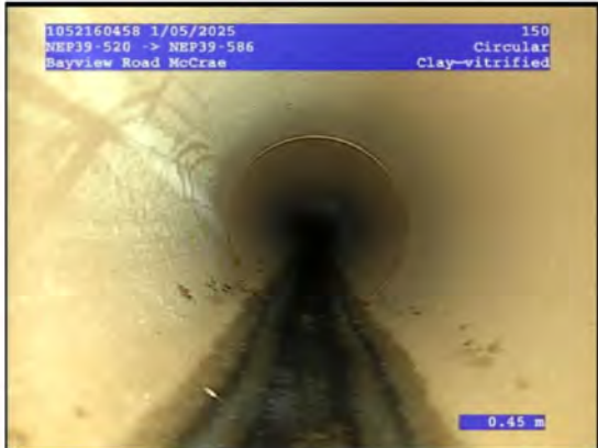
1, 00:00:27, 0.45 Water flow at constant depth, turbid or discoloured water, <5%
