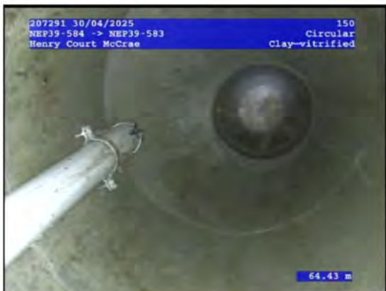
11, 00:30:07, 64.43 Finish node, maintenance hole, Nodename:, NEP39-583
