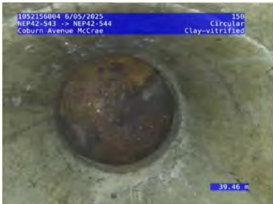
7, 00:17:54, 39.46 Finish node, maintenance hole, Nodename:, NEP42-544
