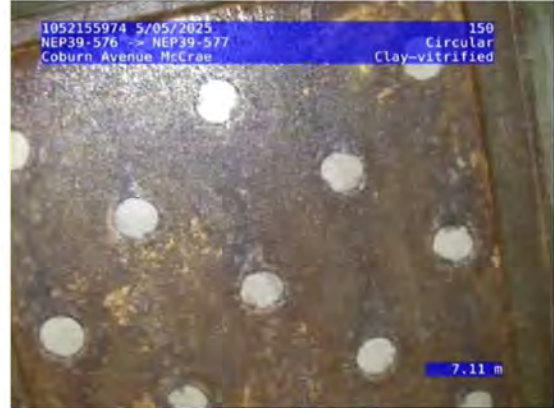
2, 00:03:27, 7.11 Finish node, maintenance hole, Nodename:, NEP39-577
