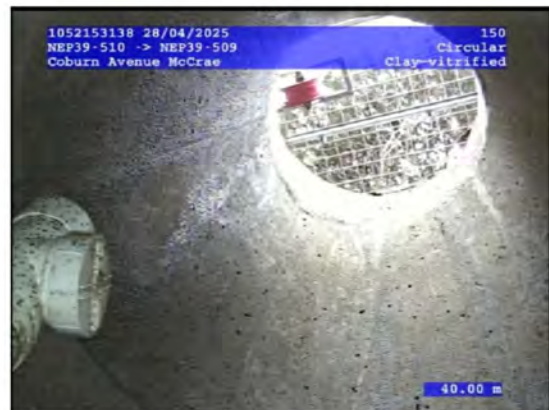
4, 00:13:39, 40.00 Finish node, maintenance hole, Nodename:, NEP39-509
