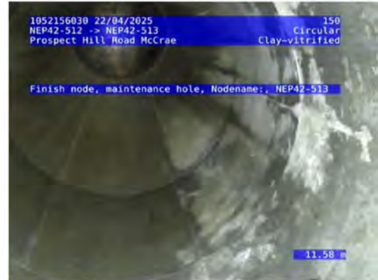
2, 00:04:24, 11.58 Finish node, maintenance hole, Nodename:, NEP42-513
