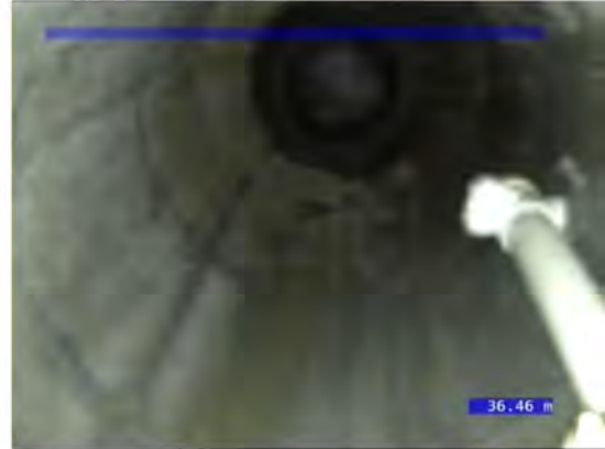
6, 00:11:41, 36.46 Finish node, maintenance hole, Nodename:, NEP42-514
