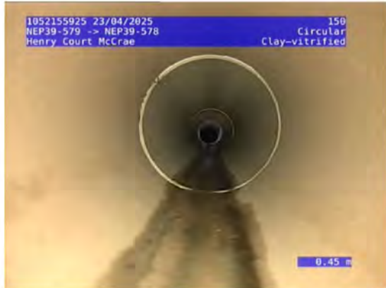
1, 00:00:22, 0.45 Water flow at constant depth, turbid or discoloured water, <5%
