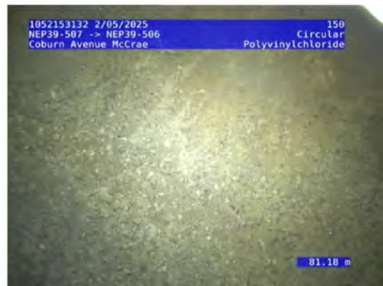
8, 00:19:40, 81.18 Finish node, maintenance hole, Nodename:, NEP39-506, reference: drop pipe
