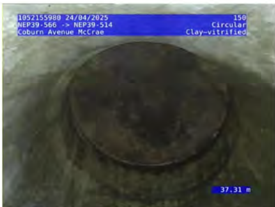
7, 00:14:17, 37.31 Finish node, maintenance hole, Nodename:, NEP39-514
