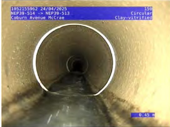
1, 00:00:26, 0.45 Water flow at constant depth, turbid or discoloured water, <5%
