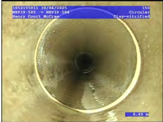
1, 00:00:00, 0.45 Water flow at constant depth, turbid or discoloured water, <5%
