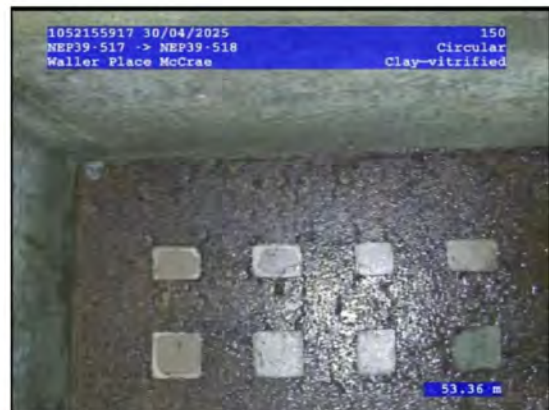
16, 00:21:20, 53.36 Finish node, maintenance hole, Nodename: NEP39-518
