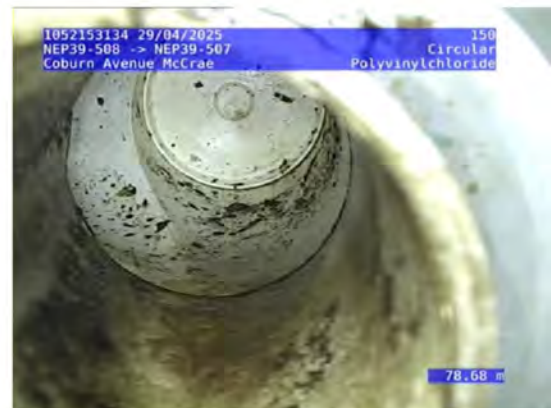
16, 00:19:28, 78.68 Junction, unlined, open, Height/Diameter (mm): 100 at 12 o'clock / 150 junction with 100mm connection
