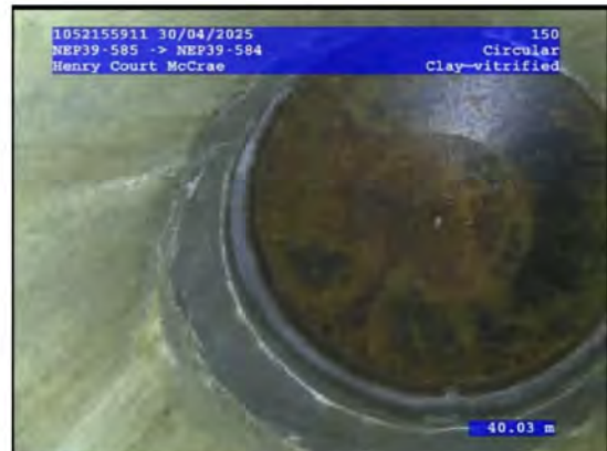
16, 00:19:47, 40.03 Finish node, maintenance hole, Nodename: NEP39-584
