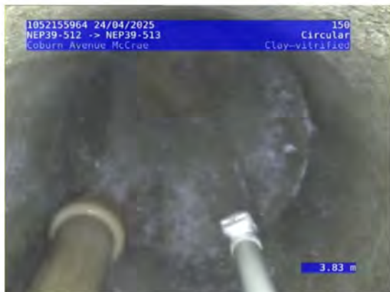
3, 00:02:33, 3.83 Finish node, maintenance hole, Nodename:, NEP39-513
