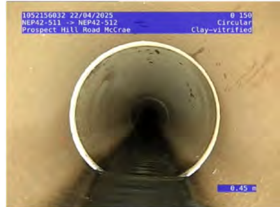
2, 00:00:36, 0.45 Water flow at constant depth, turbid or discoloured water, <5%
