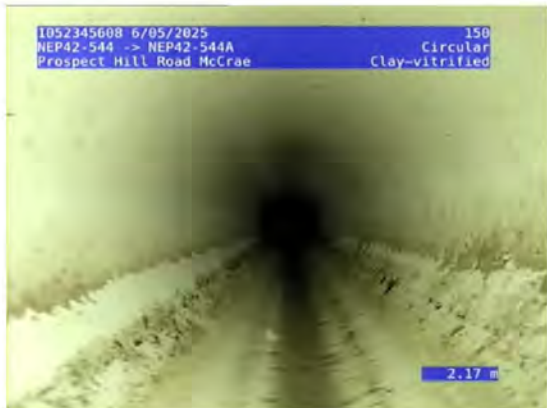
3, 00:05:45, 2.03 Inspection (survey) abandoned, obstruction / camera unable to drive further, but line visible clear and working
