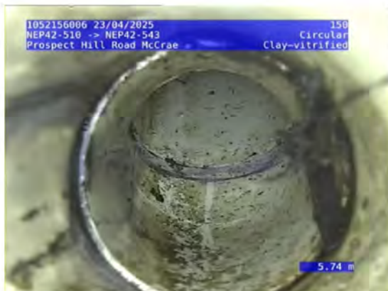
3, 00:02:14, 5.74 Junction, unlined, open, Height/Diameter (mm): 100 at 9 o'clock
