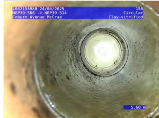
2, 00:02:48, 5.60 Junction, unlined, open, Height/Diameter (mm): 100 at 12 o'clock
