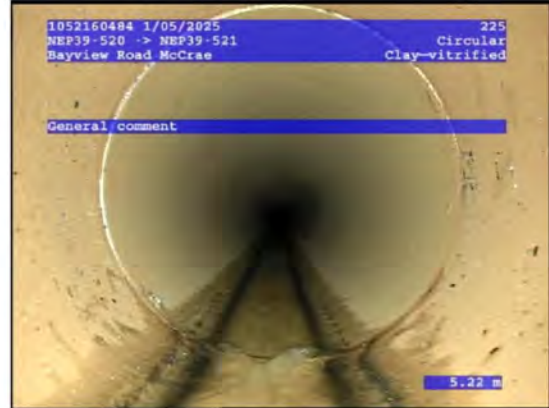
2, 00:09:16, 5.23 General comment / crawler is driving slow due to incline of pipeline.
