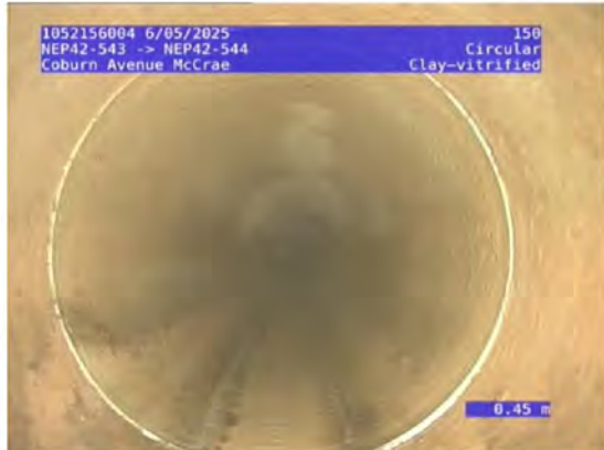
1, 00:00:25, 0.45 Water flow at constant depth, turbid or discoloured water, <5%
