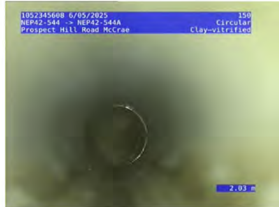
2, 00:05:45, 2.03 Inspection (survey) abandoned, obstruction / camera unable to drive further, but line visible clear and working
