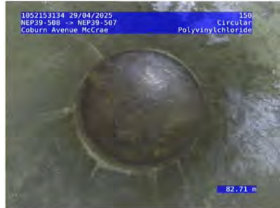
18, 00:21:24, 82.72 Finish node, maintenance hole, Nodename:, NEP39-507
