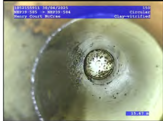
2, 00:06:57, 15.67 Junction, unlined, open, Height/Diameter (mm): 100 at 12 o'clock
