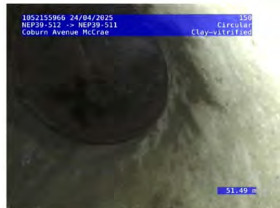
4, 00:16:46, 51.49 Finish node, maintenance hole, Nodename:, NEP39-511
