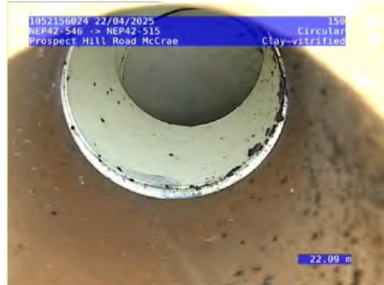
2, 00:07:05, 22.09 Junction, unlined, open, Height/Diameter (mm): 100 at 2 o'clock
