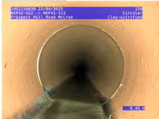
1, 00:00:21, 0.45 Water flow at constant depth, turbid or discoloured water, <5%
