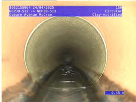
1, 00:00:23, 0.45 Water flow at constant depth, turbid or discoloured water, 5-10%
