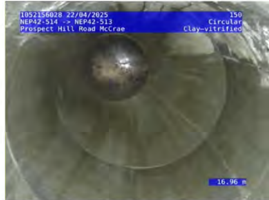
2, 00:06:52, 16.96 Finish node, maintenance hole, Nodename:, NEP42-513
