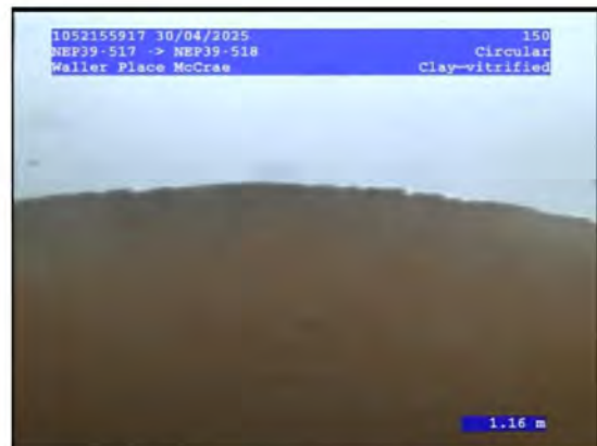
4, 00:01:53, 1.16 Change of conduit material. New material, Vitrified clay, at joint
