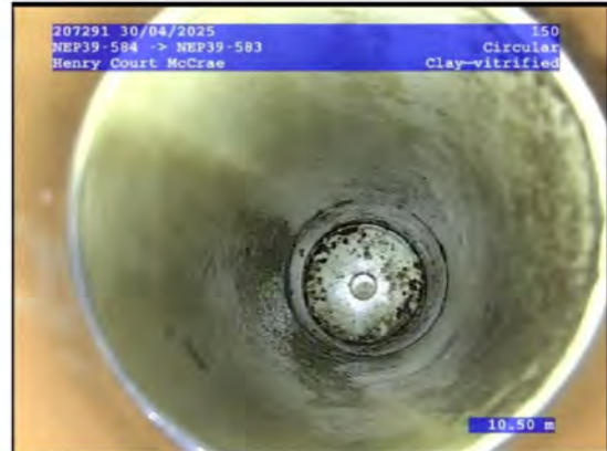
2, 00:05:23, 10.50 Junction, unlined, open, Height/Diameter (mm): 100 at 12 o'clock
