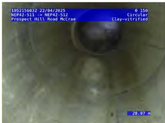
7, 00:11:23, 28.97 Finish node, maintenance hole, Nodename:, NEP42-511
