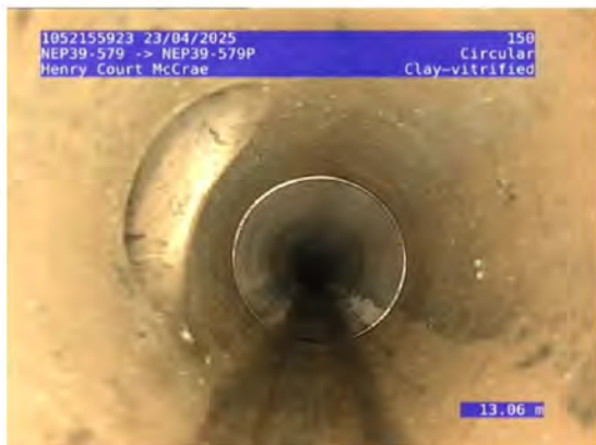
7, 00:06:53, 13.06 Junction, unlined, open, Height/Diameter (mm): 100 at 9 o'clock
