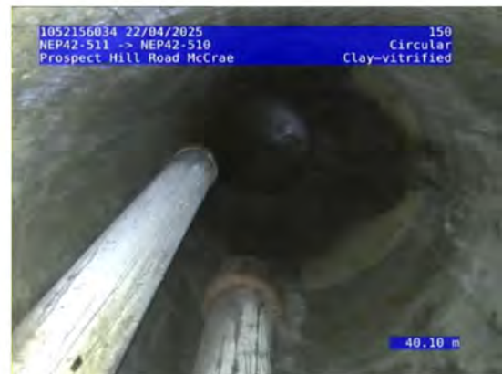
4, 00:13:58, 40.10 Finish node, maintenance hole, Nodename:, NEP42-510
