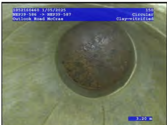
3, 00:02:04, 3.20 Finish node, maintenance hole, Nodename:, NEP39-587
