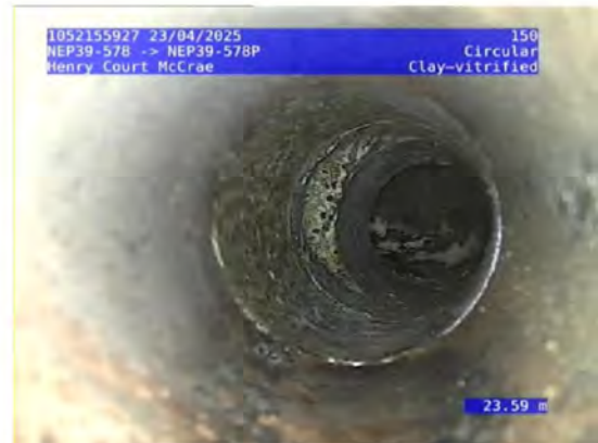
4, 00:08:21, 23.59 Junction, unlined, open, Height/Diameter (mm): 100 at 2 o'clock
