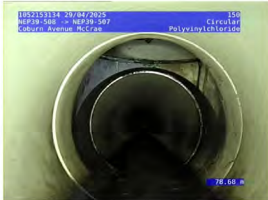
17, 00:19:28, 78.68 Junction, unlined, open, Height/Diameter (mm): 100 at 12 o'clock / 150 junction with 100mm connection
