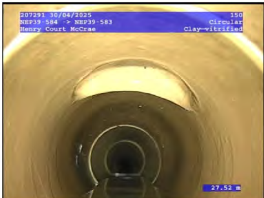
7, 00:12:24, 27.52 Junction, unlined, open, Height/Diameter (mm): 100 at 12 o'clock
