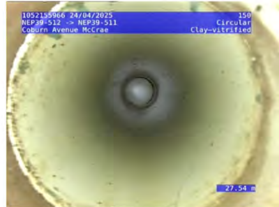
2, 00:09:04, 27.54 Junction, unlined, open, Height/Diameter (mm): 100 at 12 o'clock
