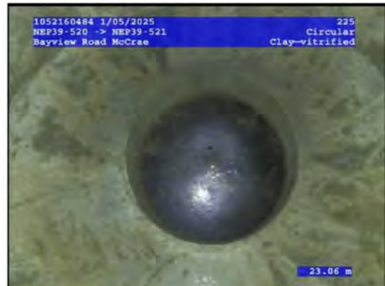
4, 00:47:55, 23.06 Finish node, maintenance hole, Nodename:, NEP39-521
