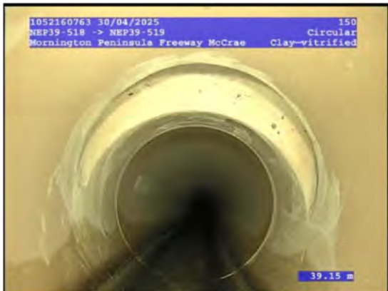
3, 00:13:28, 39.15 Junction, unlined, closed, Height/Diameter (mm): 150 at 12 o'clock
