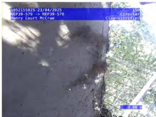
3, 00:03:02, 3.80 Finish node, maintenance hole, Nodename:, NEP39-578
