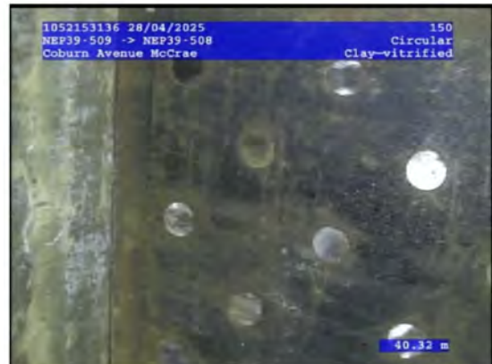
8, 00:15:53, 40.32 Finish node, maintenance hole, Nodename:, NEP39-508
