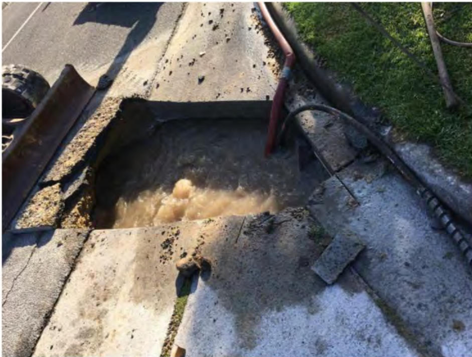
Figure 22: Photograph from SEW taken on 15 November 2022 (approximately), showing detail of water beneath concrete pavement construction prior to repair, being pumped out.
