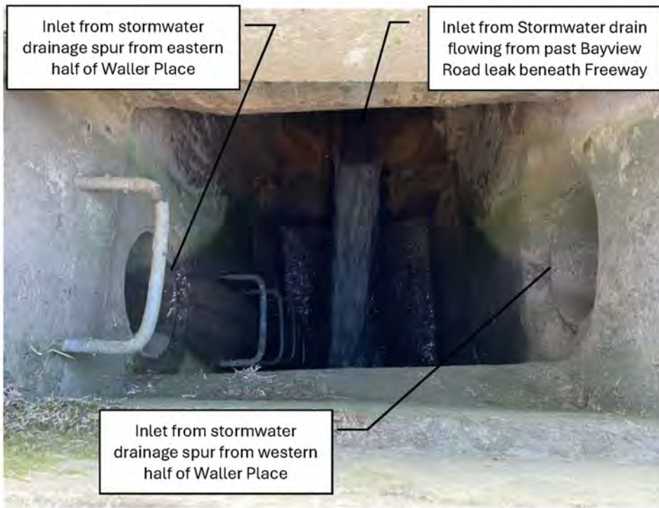
Figure 41: Photograph supplied by SEW, taken on 30 December 2024, showing water flowing into pit opposite 6 Waller Place
