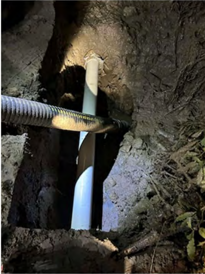
Figure 47: Provided by SEW, understood to have been taken on 1 January 2025, at the Bayview Road leak site showing exposure of pipe. Indicating the fracture is at the bottom of the pipe.
