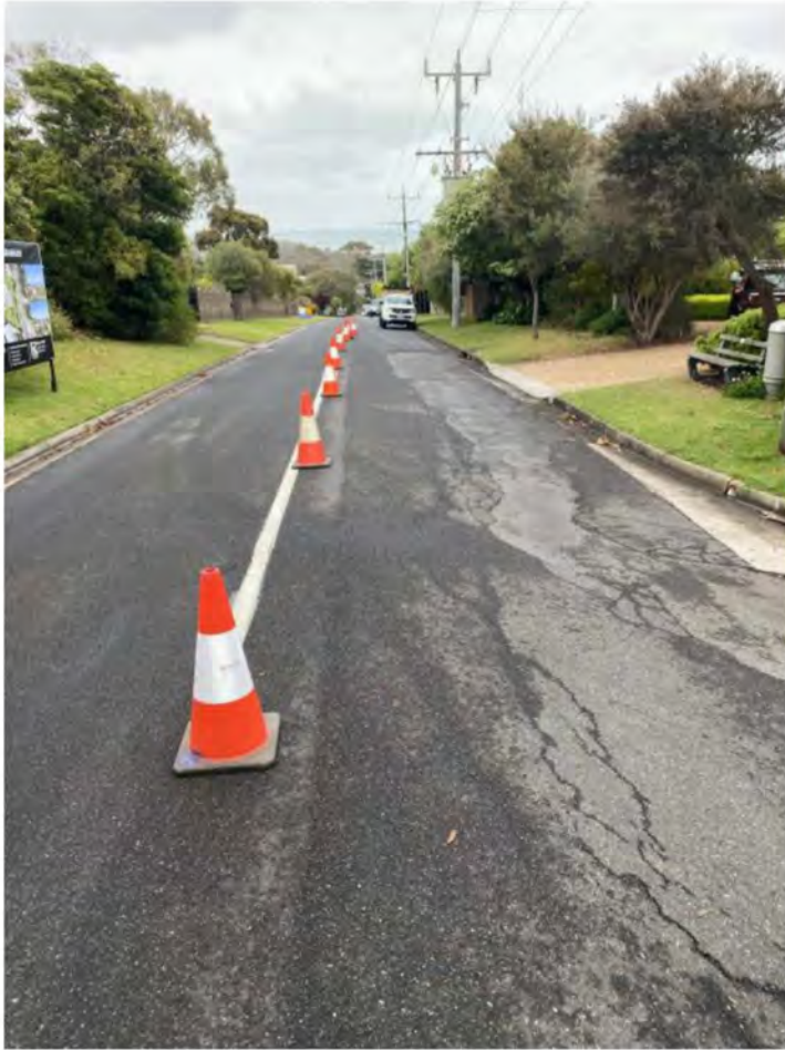
Figure 28: Photograph from SEW taken on 29 November 2023 (approximately), looking west along Coburn Avenue from junction with Prospect Hill Road showing condition of pavement prior to repair works.
