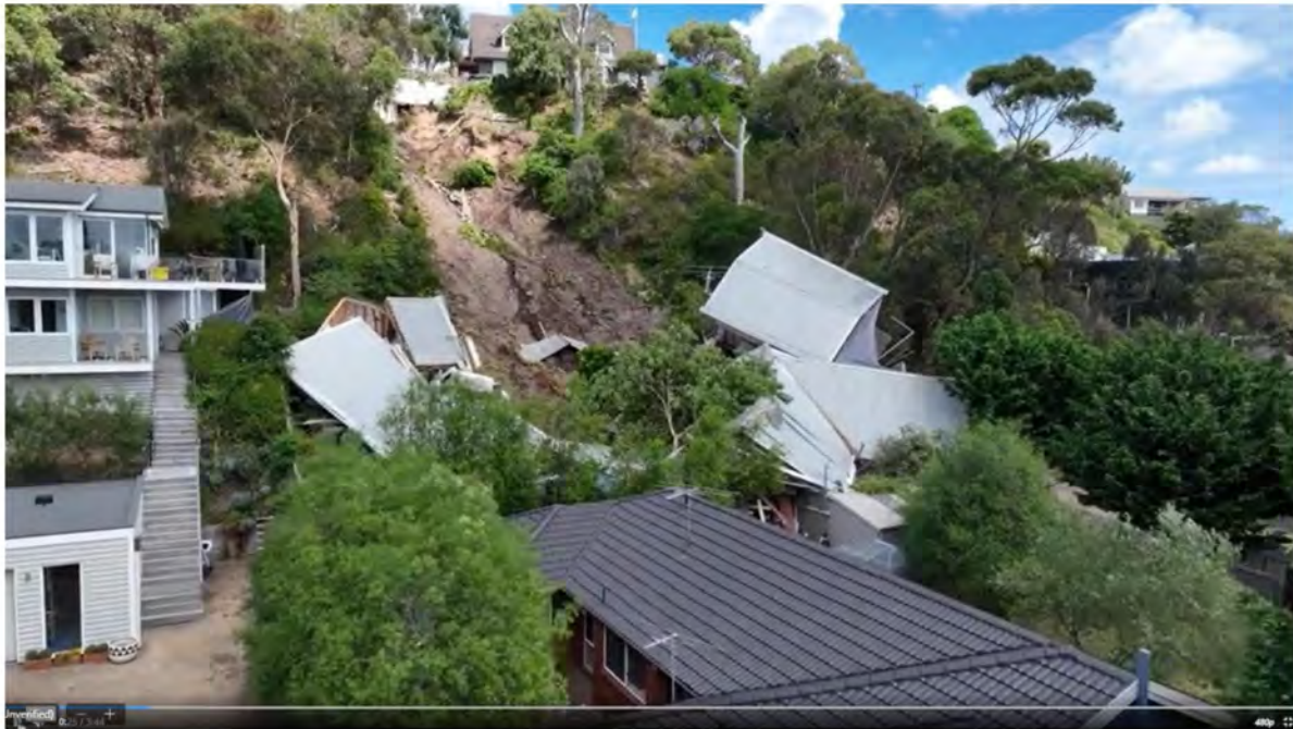
Figure 10: Drone footage taken from toe of slope failure showing the gully, denuded by slipping debris from upslope.
