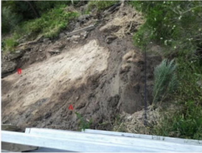
Picture 6 – looking North over timber stairs showing seeps A and B after landslip November 2022
