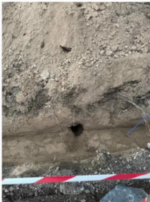
Picture 8 - Void discovered during earthworks to install drainage and new kerb on View Point road
