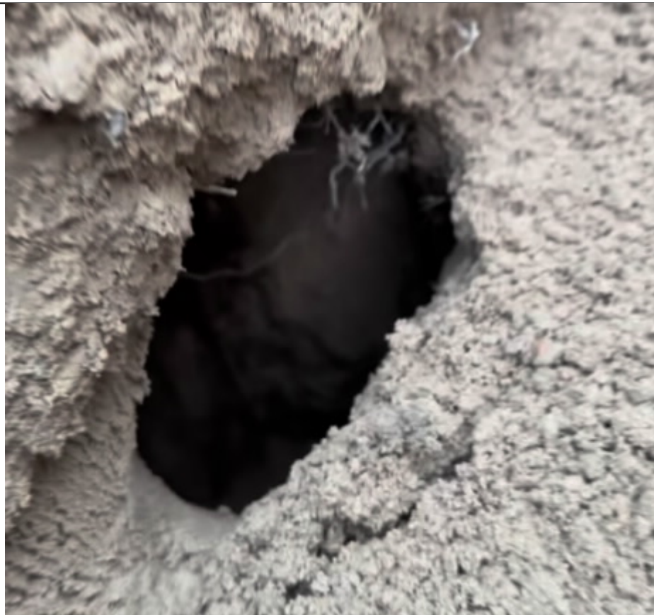
Fig 7: Still image showing void, taken from a video provided by Gerry Borghesi during Storm Water upgrade.
