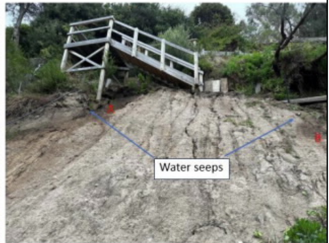
Picture 7 – looking South over landslide showing seeps A and B flanking the landslide
