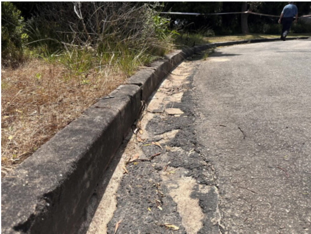
Figure 8: Cracks and patching along the kerb on View Point Road
