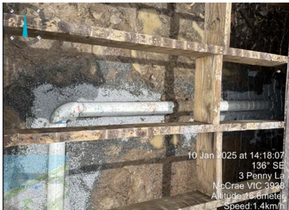
Photo 1: Initial Drainage diversion
