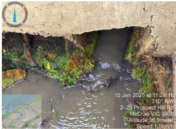
Photo 9: Corner of View Point road and Prospect Hill Road stormwater pit no red dye.
