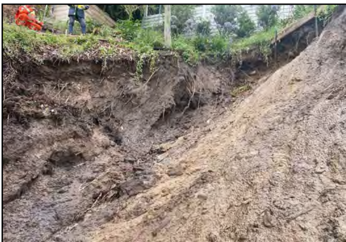
Photo 1 - Seepage at XW Granite contact and partially saturated fills of headscarp (06/01/2025)
