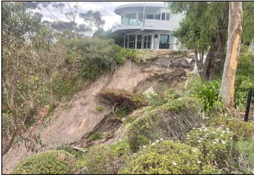
Photo 15A - Seepage line of Eastern flank (30/01/2025)
