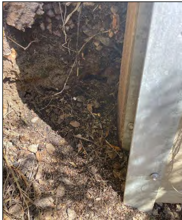
Photo 14 - Saturated soils adjacent to retaining wall at stairs on 10-12 View Point Road (24/01/2025)
