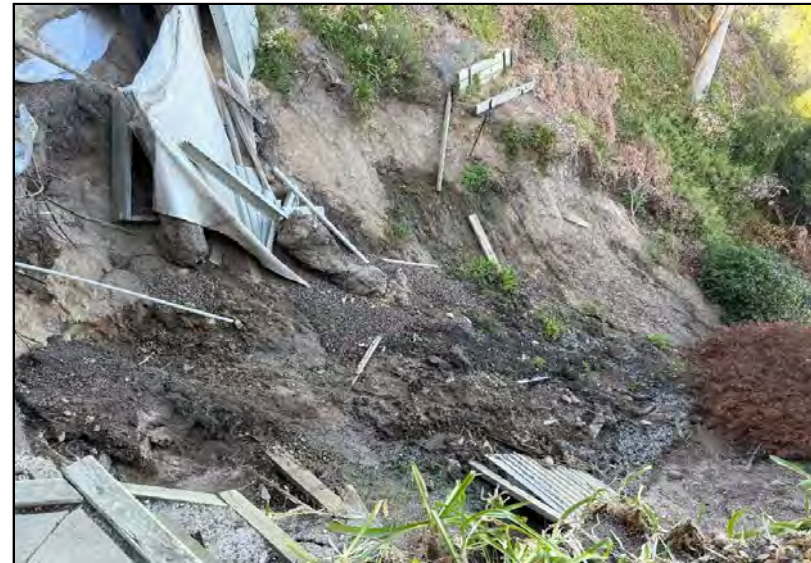
Photo 26B - Seepage line of Western flank (28/02/2025)
