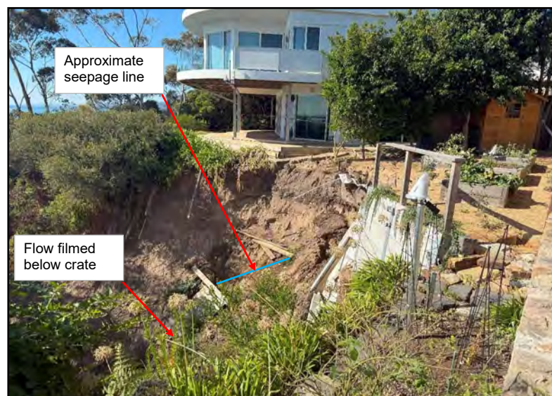
Photo 34A - Seepage line of Eastern flank (10/04/2025)
