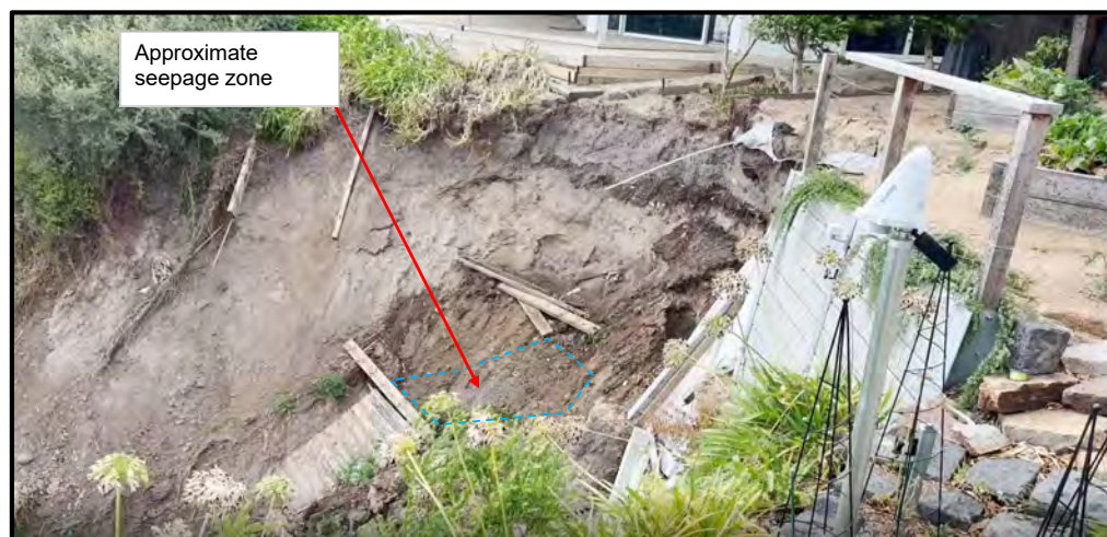
Photo 31A - Seepage zone of Eastern flank (20/03/2025)
