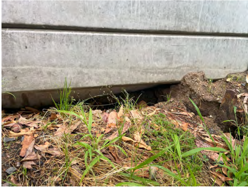
Inset 50: 2024 RW on 6 January 2025. Refer to Figure 9 for tension crack location in plan. I note that the concrete panels are 200 mm in height
