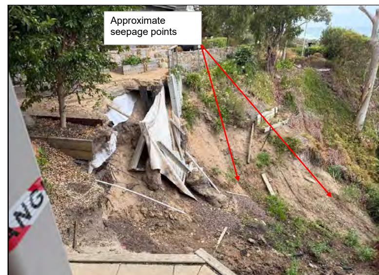
Photo 31B - Seepage line of Western flank (20/03/2025)
