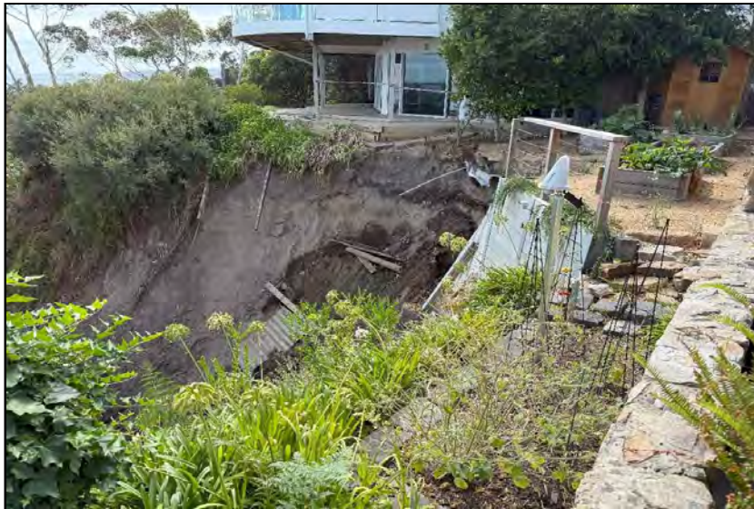
Photo 26A - Seepage line of Eastern flank (28/02/2025)
