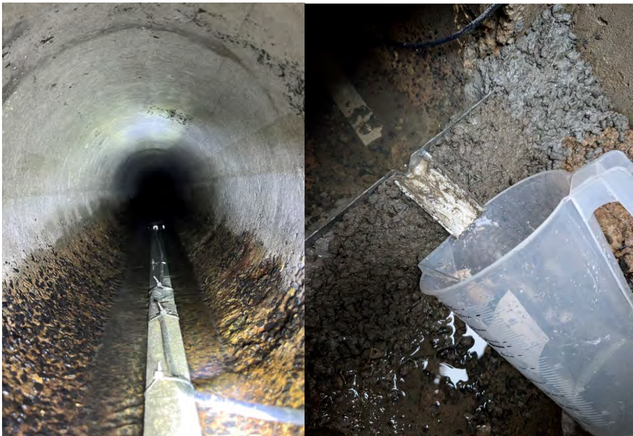
Inset 36: Installation of Starflow sensor (left) and flow measurement from weir (right).
