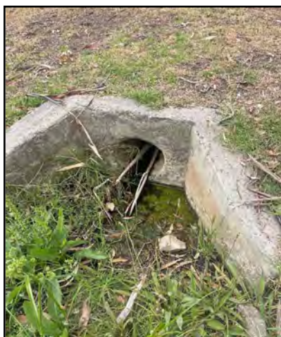
Photo 18 - Inferred base flows in reserve near 44 The Boulevard (30/01/2025)
