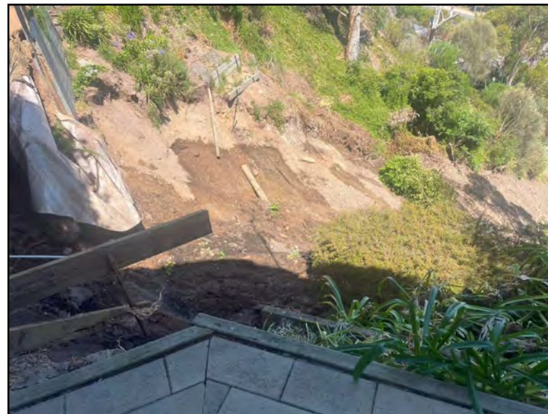
Photo 11B - Seepage line of Western flank (21/01/2025)
