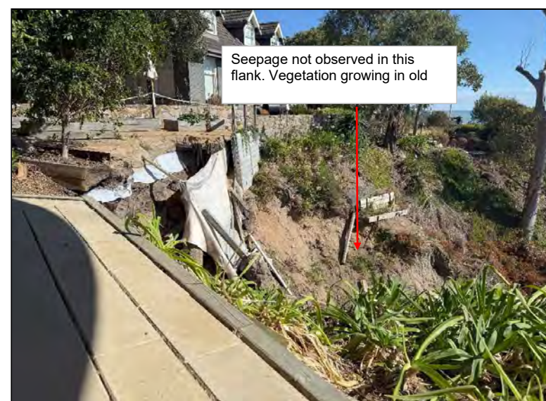
Photo 34B - Seepage line of Western flank (10/04/2025)
