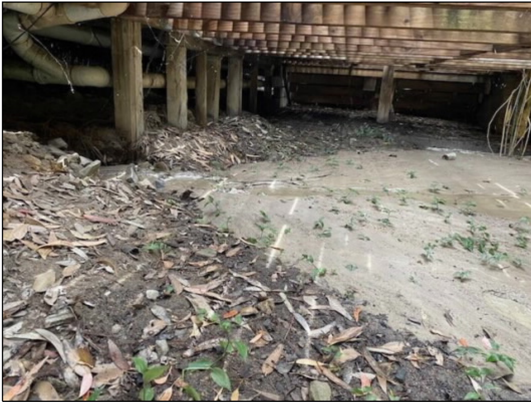
Photograph 6: Deposited sediment under 3 Penny Lane from streamflow
