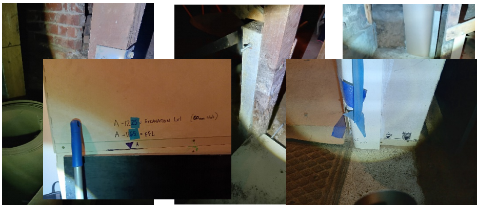
Figure 4 - Notes regarding proposed floor levels for concrete and excavation
