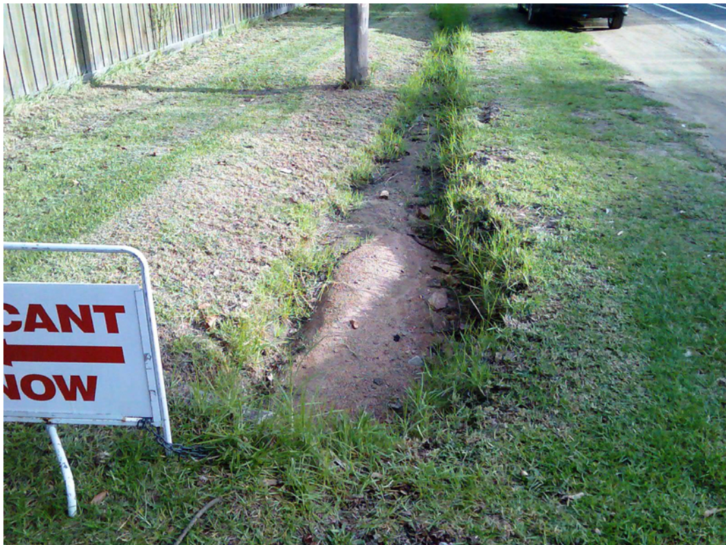
Plate 3.I: Blocked street drainage on Point Nepean Road
