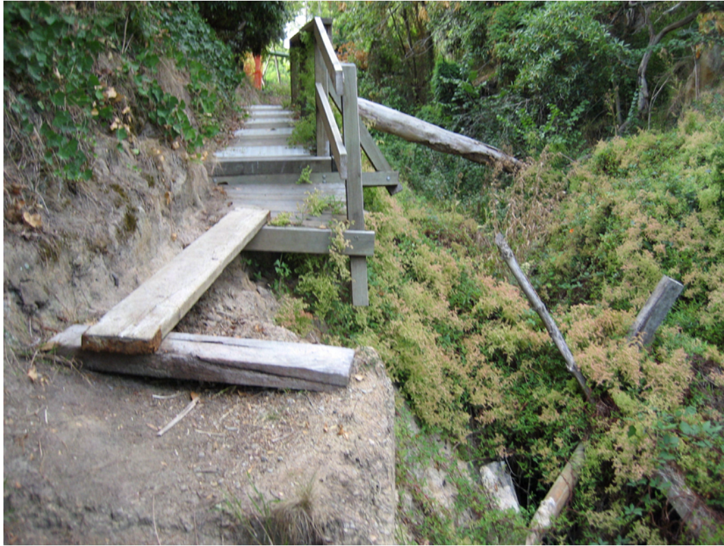
Plate 3.E: Collapsed Boardwalk in vicinity of Section C-C'
