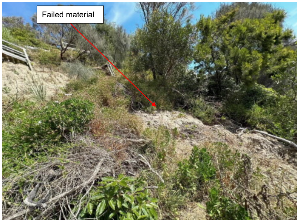
Photo 4 - Failed material still on slope
