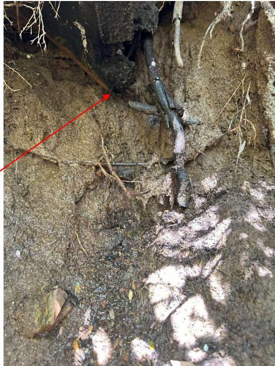
Photo 6 - Groundwater seepage
