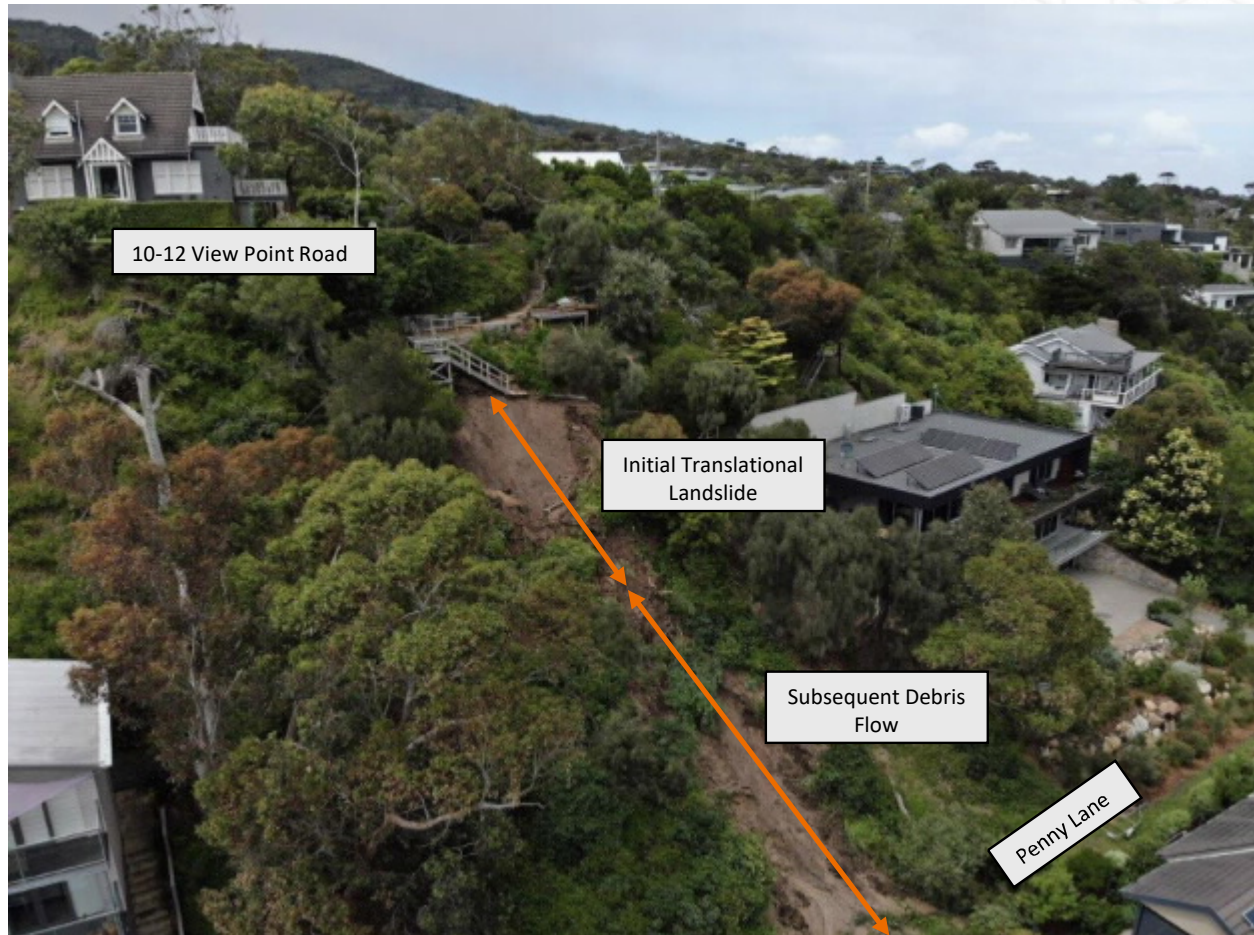
Figure 3-1: Oblique view of landslides
