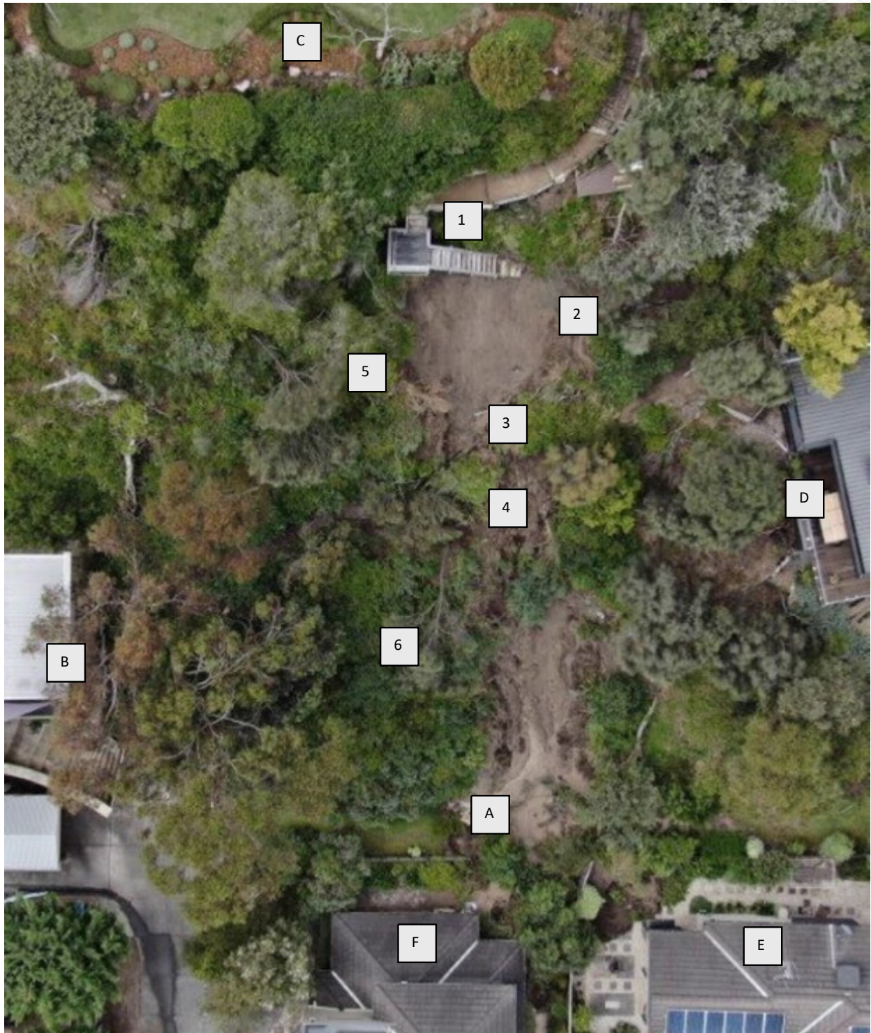
Figure 5-1: Potential Landslide Hazards and Properties at Risk
