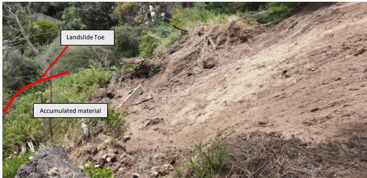
Figure 4-3: Accumulation zone of landslide
