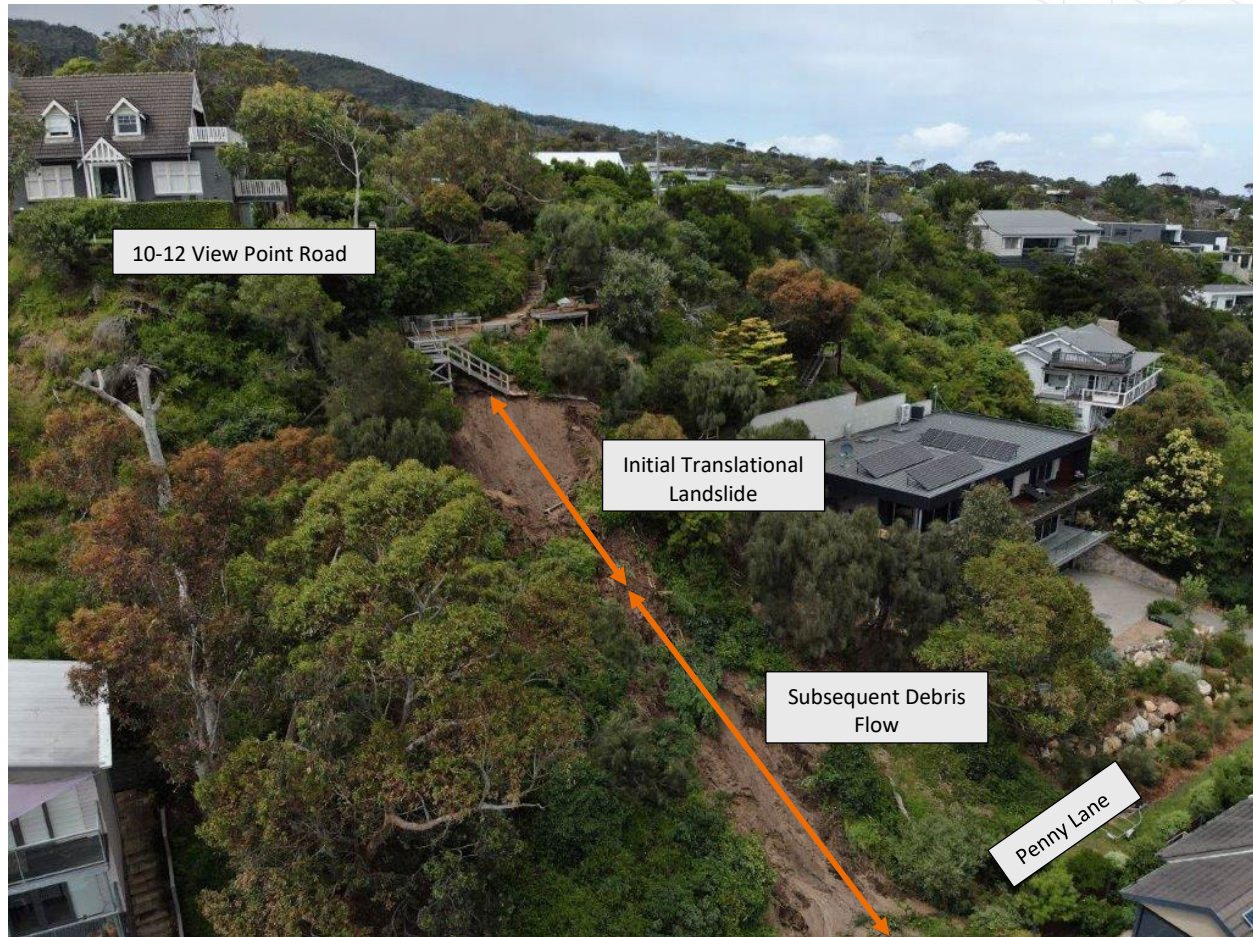
Figure 3-1: Oblique view of landslides
