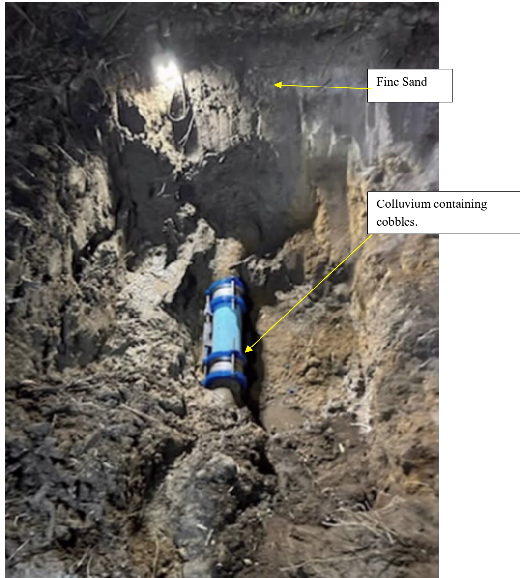
Figure 8.17 Photo of pipe repair (SME.0001.0001.0047).
