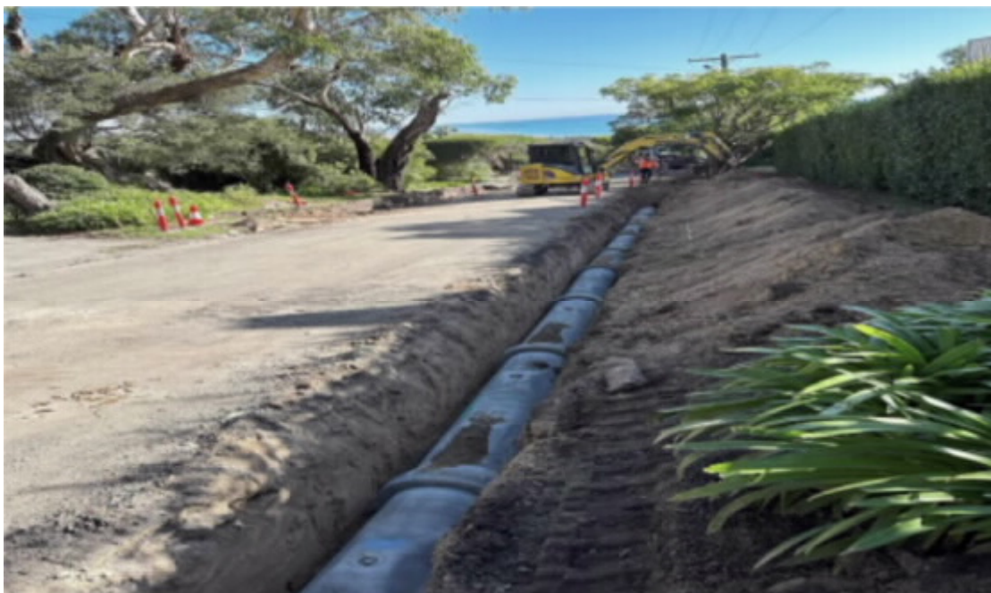
Figure 7.17 Stormwater trench backfill (RES.0001.0003.0001).
