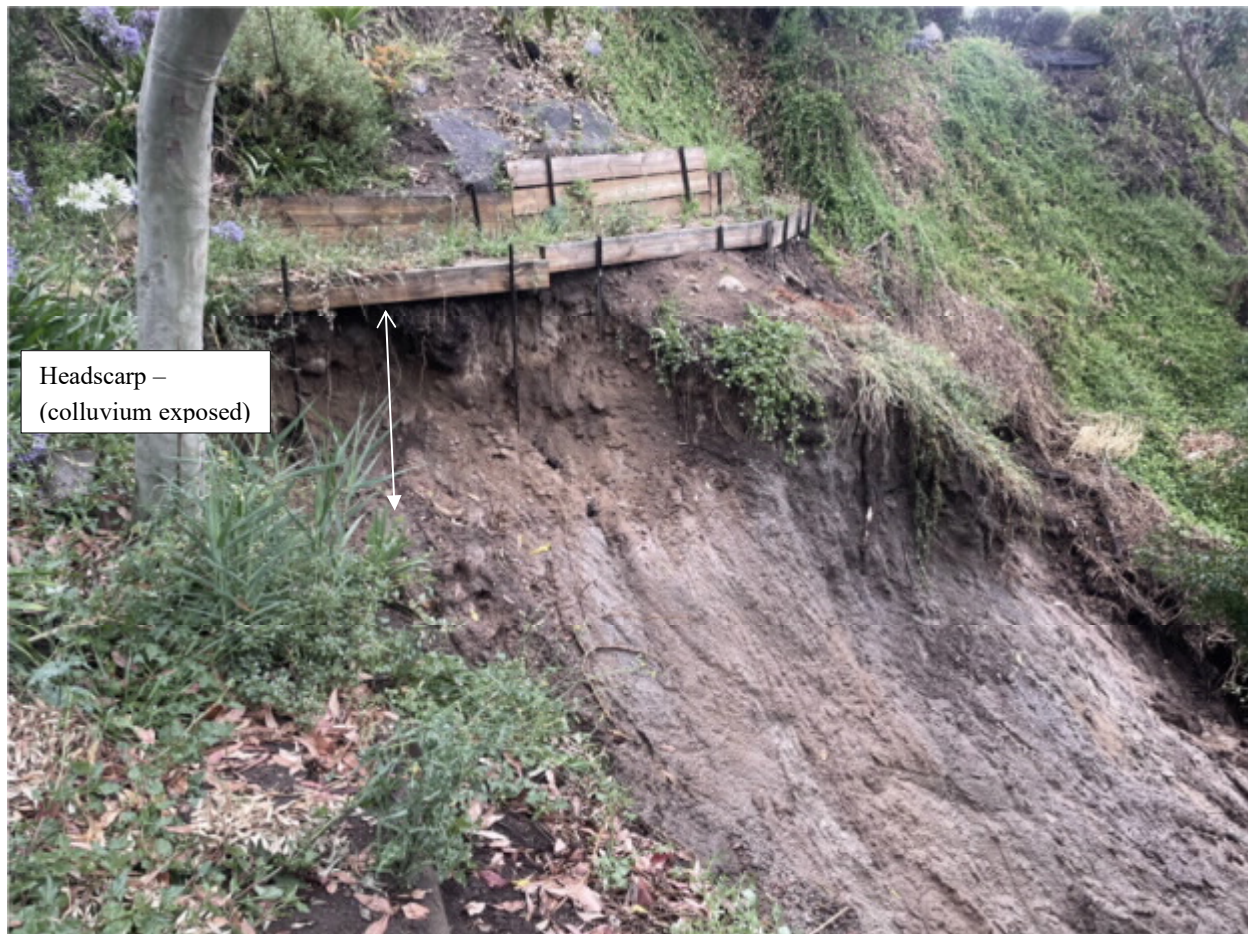
Figure 8.1 Headscarp following 5 January landslide.
