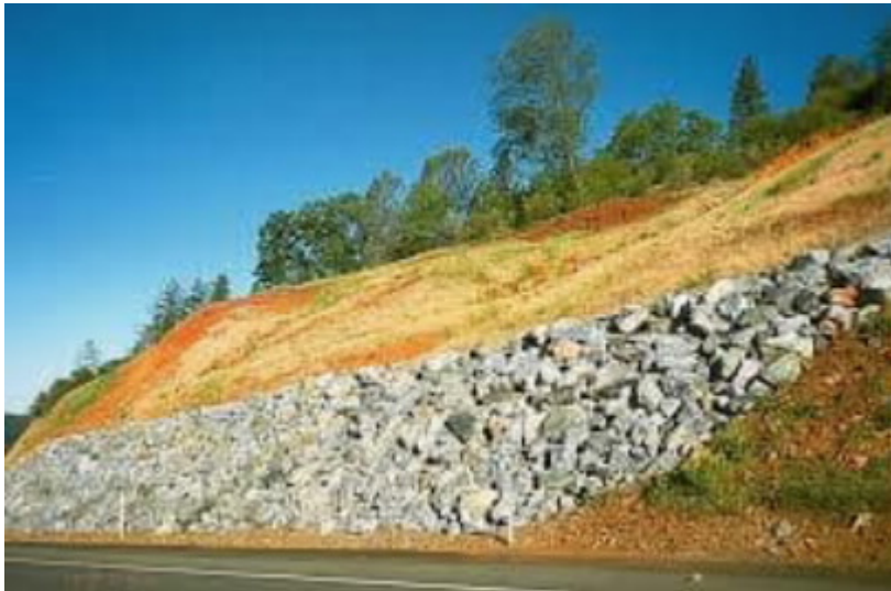
Figure 9.3 Image of landslide reinstated using rockfill 19 .
