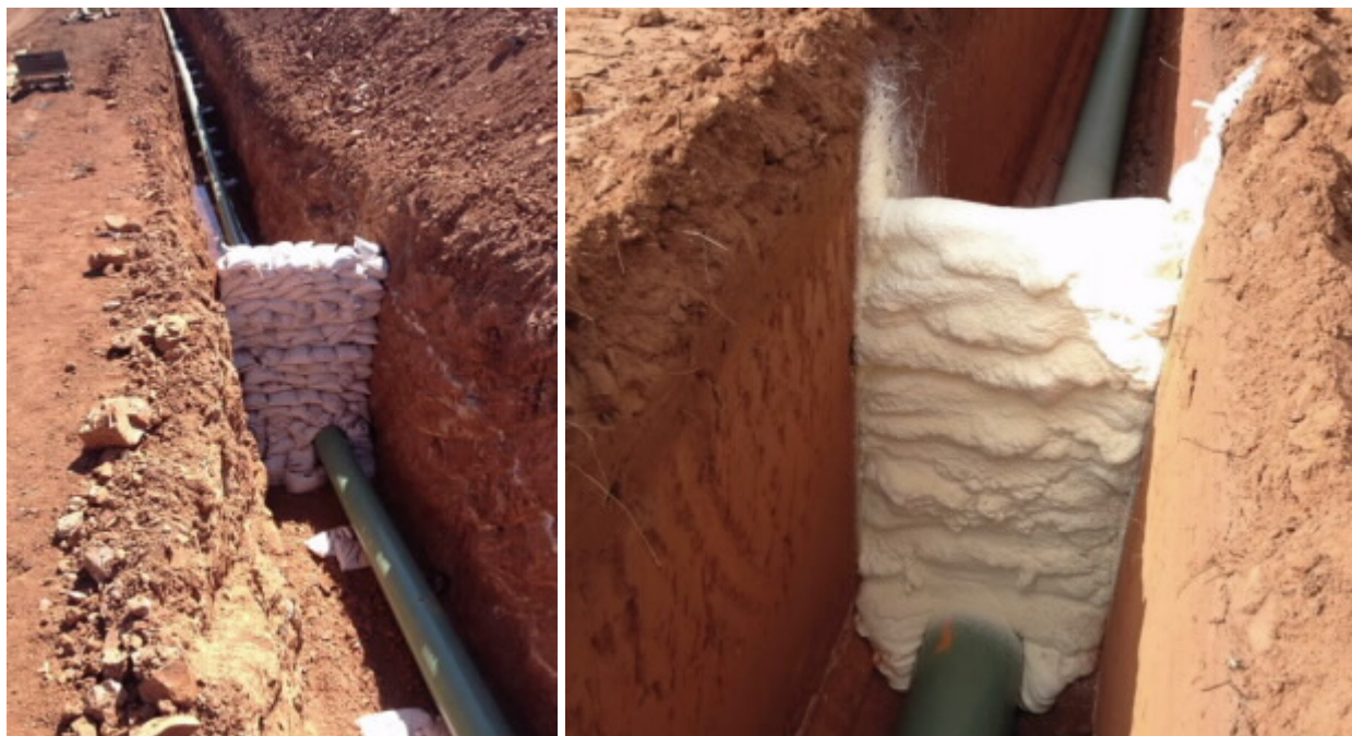
Figure 9.8 Example of trench stops using sandbags (left 20 ), and foam (right 21 )
