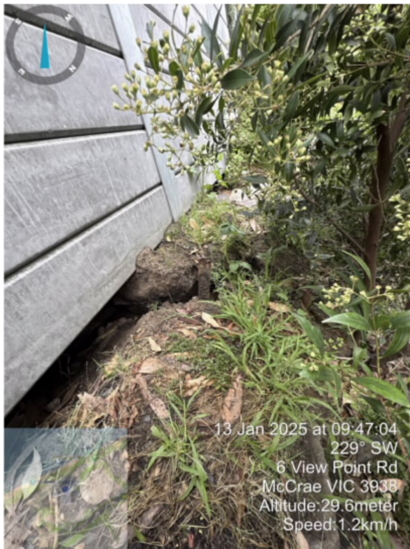
Figure 8.35 Tension Cracking at toe of retaining wall at 10-12 View Point Road (MSC.5035.0001.0033)
