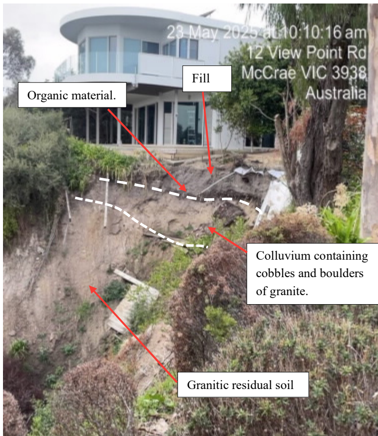
Figure 6.8 Sub-surface profile as identified within the landslide headscarp.
