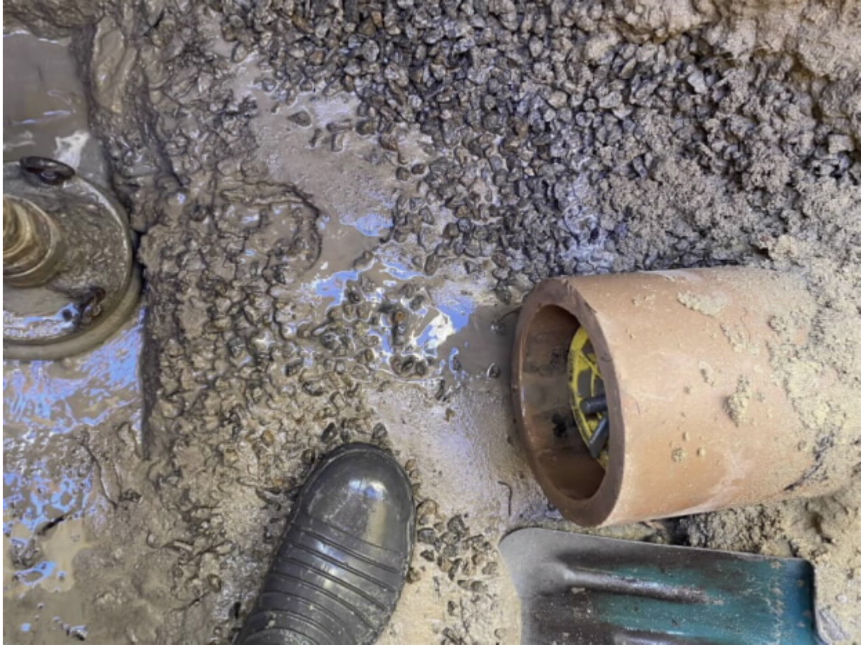
Figure 7.15 Vitreous clay sewer on gravel bed (reference SME.0001.0001.0018)
