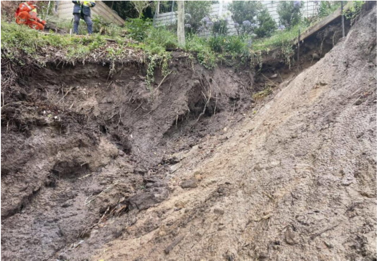
Figure 11: PSM Photograph of head-scarp, the EW granite seen in the right foreground, suggests that interface groundwater flow may be locally on an EW Granite interface, rather than on a residual interface.
