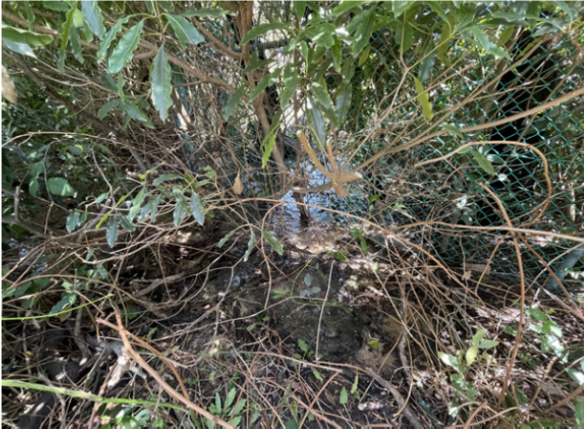
Figure 3 - Photo of the site of the Bayview Road burst, located in bushland
