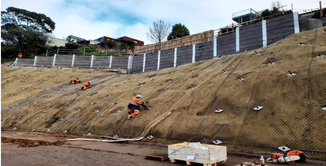
Figure 1 Soil nailed slope stabilised with Titan 40/20 Duplex hollow bar anchors
