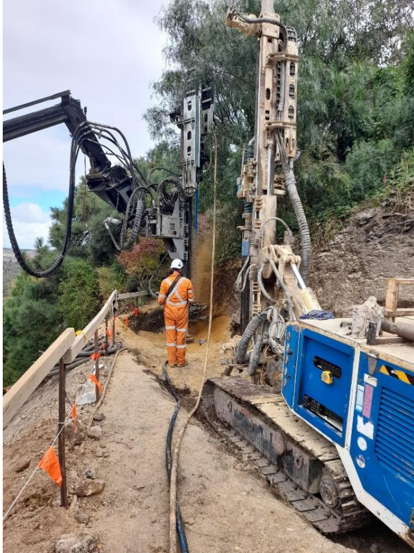
Figure 3 Titan 52/26 A Frame Micropiles for Retaining Wall Footing
