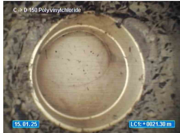
10-12 VIEW POINT ROAD MCCRAE_15.01.2025_114611_C TOO D_030.jpg, 00:04:25, 21.30 Connection, unlined, connection appears to be open, Height/Diameter (mm): 100 at 12 o'clock
