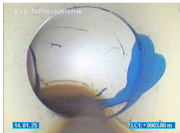
10-12 VIEW POINT ROAD MCCRAE_15.01.2025_083859_A TOO B _004.jpg, 00:05:13, 3.80 Inspection (survey) abandoned, Line deviates
