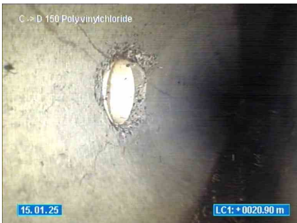
10-12 VIEW POINT ROAD MCCRAE_15.01.2025_114611_C TOO D_031.jpg, 00:04:25, 21.30 Connection, unlined, connection appears to be open, Height/Diameter (mm): 100 at 12 o'clock
