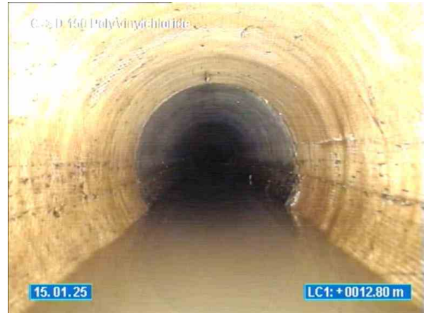
10-12 VIEW POINT ROAD MCCRAE_15.01.2025_114611_C TOO D_026.jpg, 00:04:25, 12.80 Change of conduit material. New material, Fibre reinforced plastic
