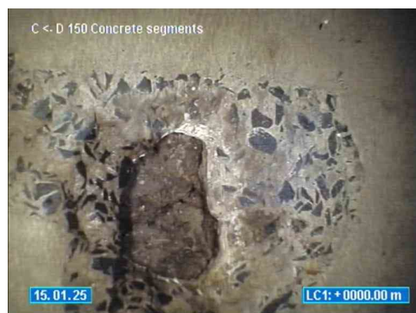
10-12 VIEW POINT ROAD MCCRAE_15.01.2025_132020_D TOO C _036.jpg, 00:33:07, 0.00 Soil visible through defect
