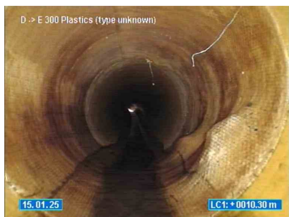
10-12 VIEW POINT ROAD MCCRAE_15.01.2025_135956_D TOO E _049.jpg, 00:01:48, 10.30 The non-structural liner has bulged (no longer attached but liner is still intact) at 4 o'clock
