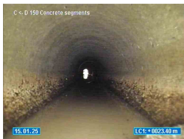
10-12 VIEW POINT ROAD MCCRAE_15.01.2025_132020_D TOO C _044.jpg, 00:33:07, 23.20 Recently cut fine roots-a relatively small number of cut minor roots remain, Obstruction: 40%, at joint from 4 o'clock to 6 o'clock
