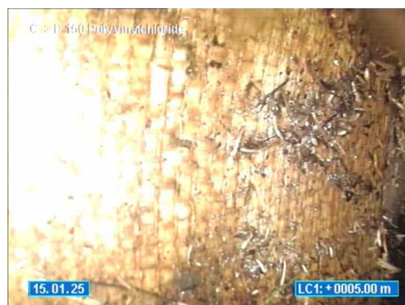
10-12 VIEW POINT ROAD MCCRAE_15.01.2025_104134_C TOO D_018.jpg, 00:03:47, 5.00 Change of conduit material. New material, Fibre reinforced plastic
