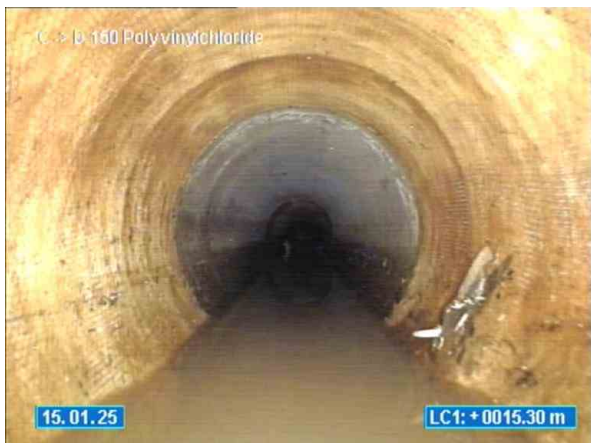
10-12 VIEW POINT ROAD MCCRAE_15.01.2025_114611_C TOO D_027.jpg, 00:04:25, 15.30 Change of conduit material. New material, Fibre reinforced plastic, at joint
