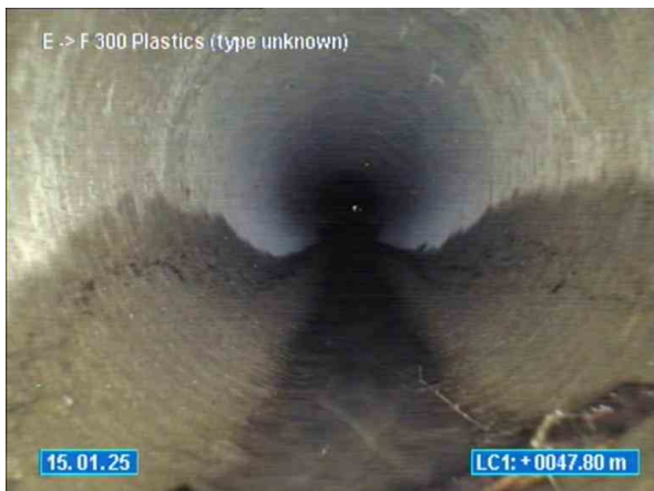
10-12 VIEW POINT ROAD MCCRAE_15.01.2025_141137_E TOO F _053.jpg, 00:05:39, 47.80 Tap roots, reduction in cross sectional area, Obstruction: 10% from 6 o'clock to 7 o'clock
