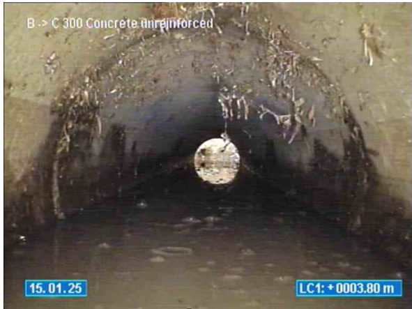
10-12 VIEW POINT ROAD MCCRAE_15.01.2025_102122_B TOO C _012.jpg, 00:03:34, 3.80 Water flow at constant depth, turbid or discoloured water, 20-25%
