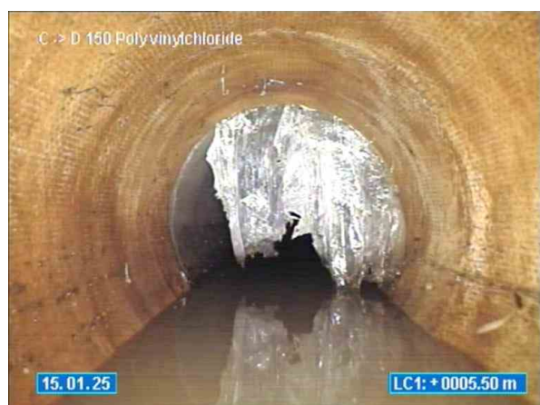
10-12 VIEW POINT ROAD MCCRAE_15.01.2025_114611_C TOO D_023.jpg, 00:04:25, 5.50 Change of conduit material. New material, Fibre reinforced cement, at joint
