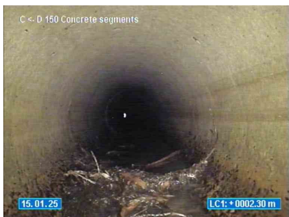
10-12 VIEW POINT ROAD MCCRAE_15.01.2025_132020_D TOO C _037.jpg, 00:33:07, 2.30 Recently cut fine roots-a relatively small number of cut minor roots remain, Obstruction: 20% from 4 o'clock to 8 o'clock
