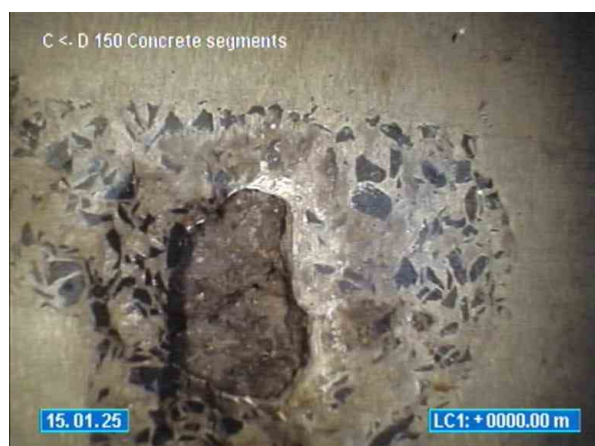
10-12 VIEW POINT ROAD MCCRAE_15.01.2025_132020_D TOO C _035.jpg, 00:33:07, 0.00 Breaking, one or more pieces of conduit are missing, length of break: 100mm from 11 o'clock to 1 o'clock
