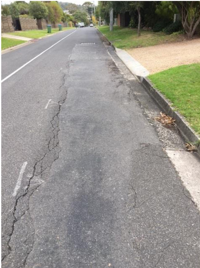
Photo 6 Photo 7 Photo 8 Photo 9 Photo 10
