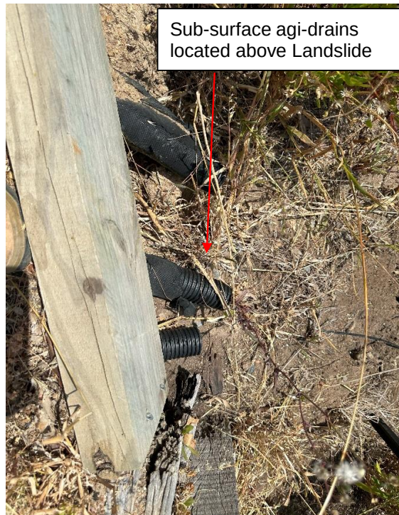
Photo 7 - Water infrastructure including water pipes (on left), and subsurface 'agi drains' (on right)
