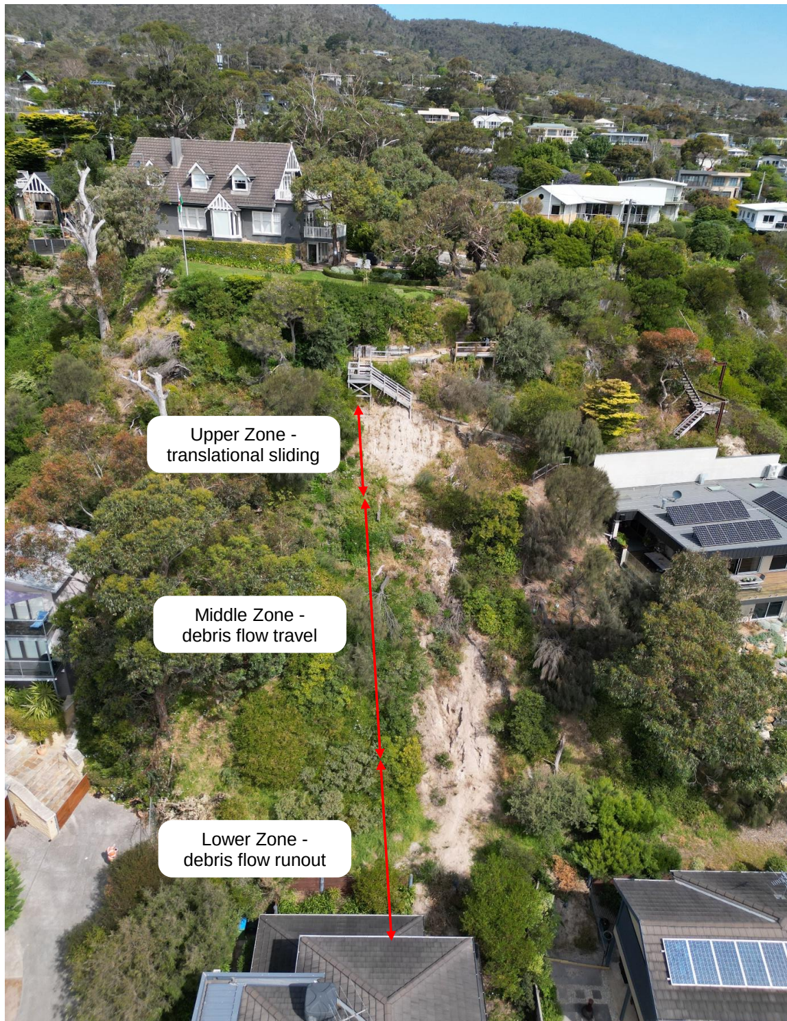
Photo 3 - Landslide Overview, with zones indicated
