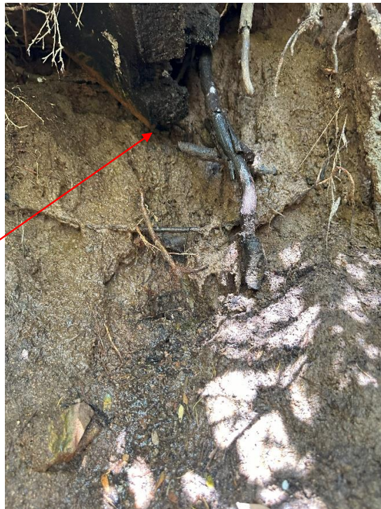
Photo 6 - Groundwater seepage
