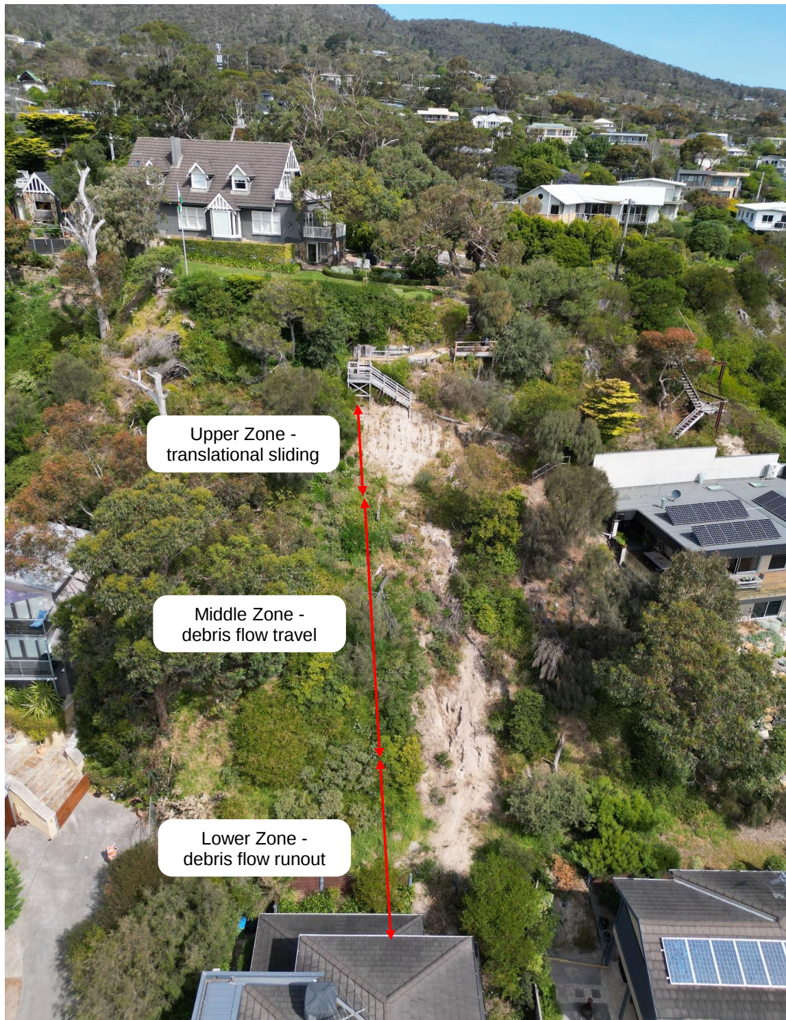
Photo 3 - Landslide Overview, with zones indicated
