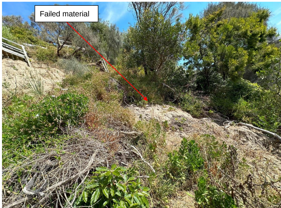
Photo 4 - Failed material still on slope
