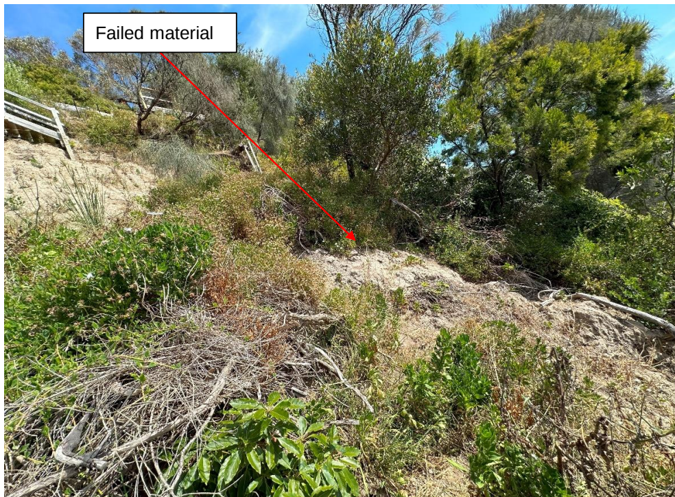
Photo 4 - Failed material still on slope
