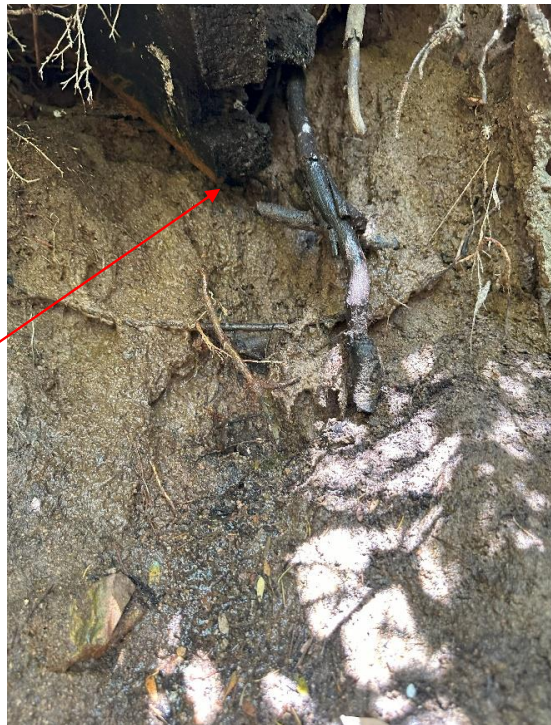
Photo 6 - Groundwater seepage
