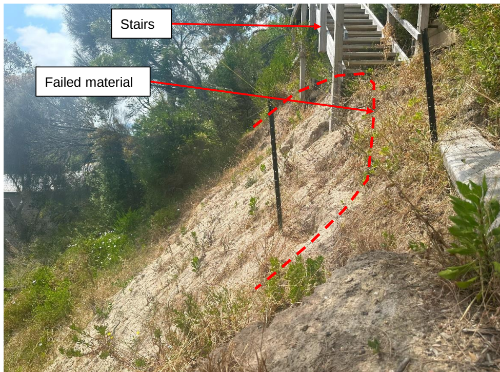
Photo 5 - Rear scarp of landslide, note lack of oversteepened backscarp
