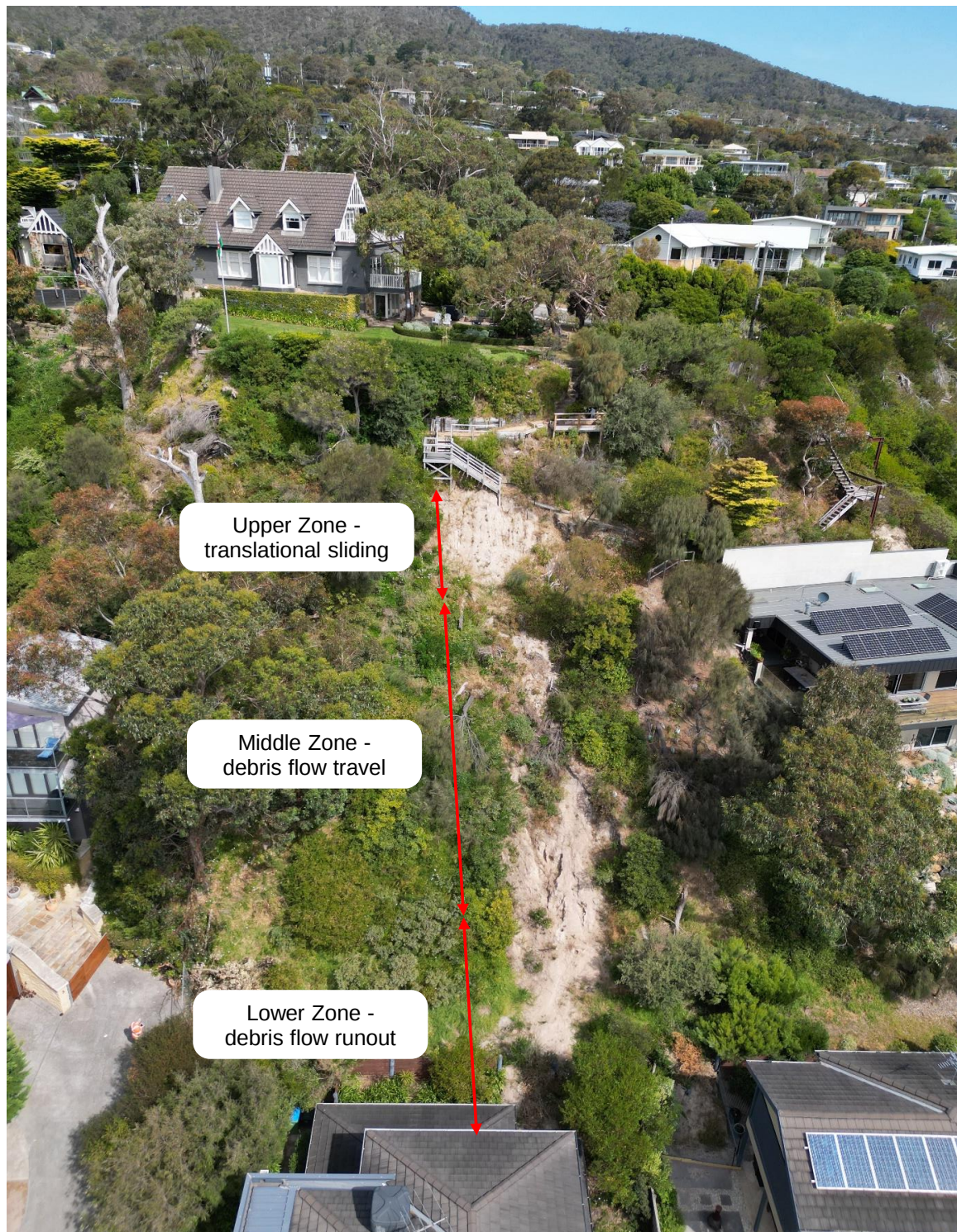
Photo 1 - Landslide Overview, with zones indicated
