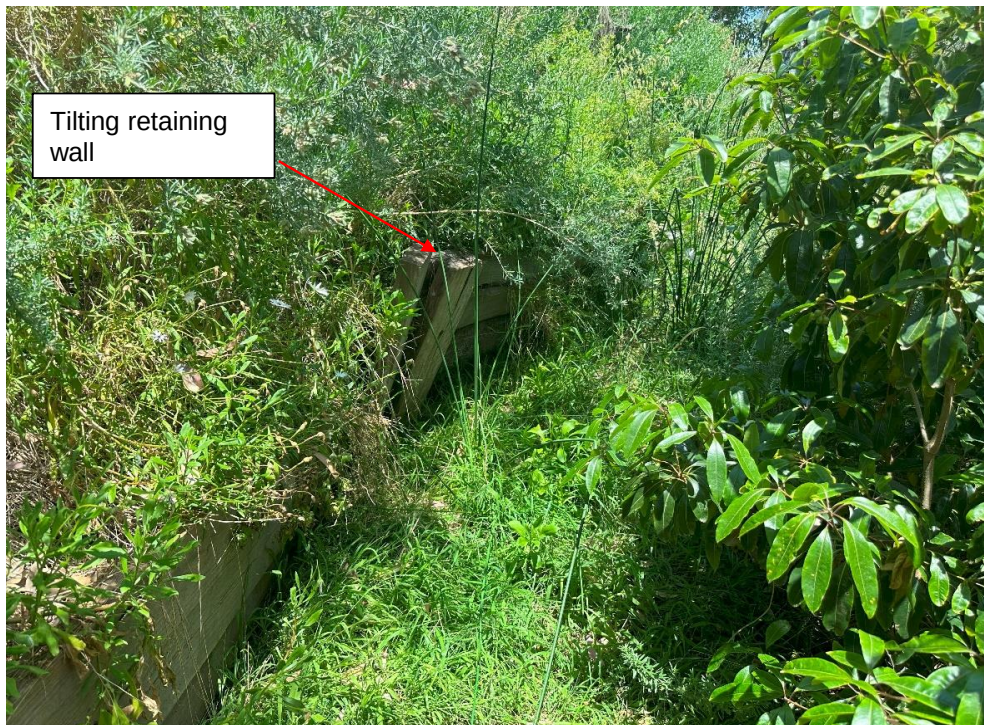
Photo 10 - Tilting retaining walls on left side of Landslide
