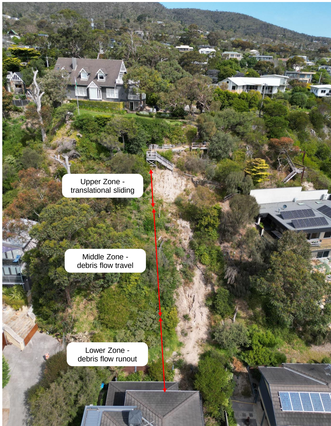
Photo 1 - Landslide Overview, with zones indicated
