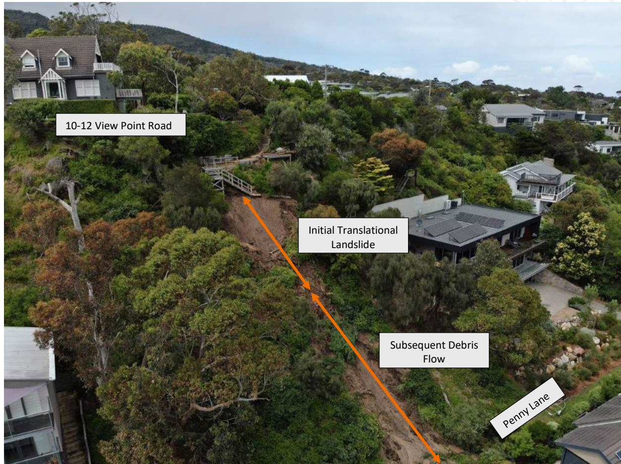
Figure 3-1: Oblique view of landslides
