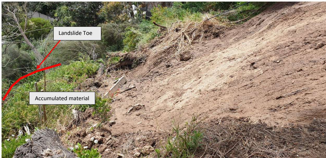
Figure 4-3: Accumulation zone of landslide
