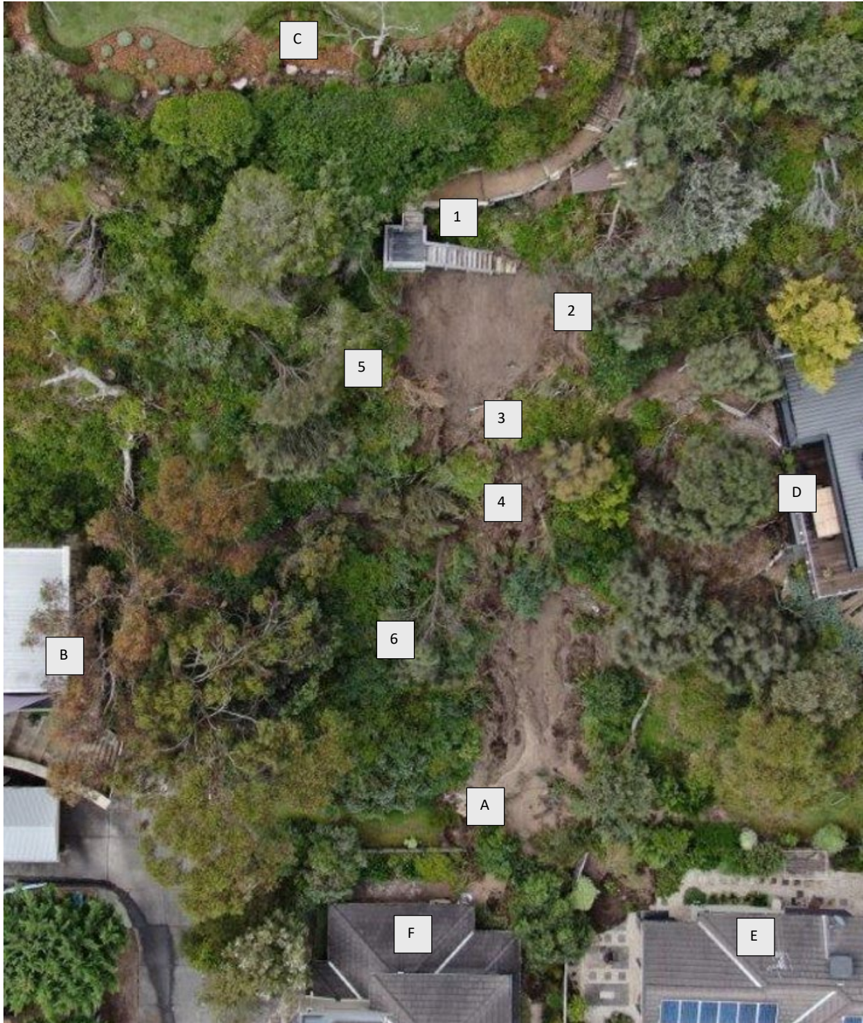
Figure 5-1: Potential Landslide Hazards and Properties at Risk
