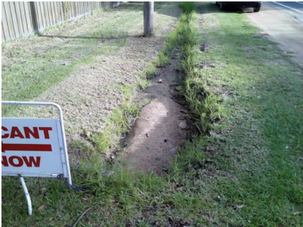
Plate 3.I: Blocked street drainage on Point Nepean Road
