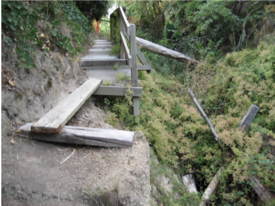
Plate 3.E: Collapsed Boardwalk in vicinity of Section C-C'
