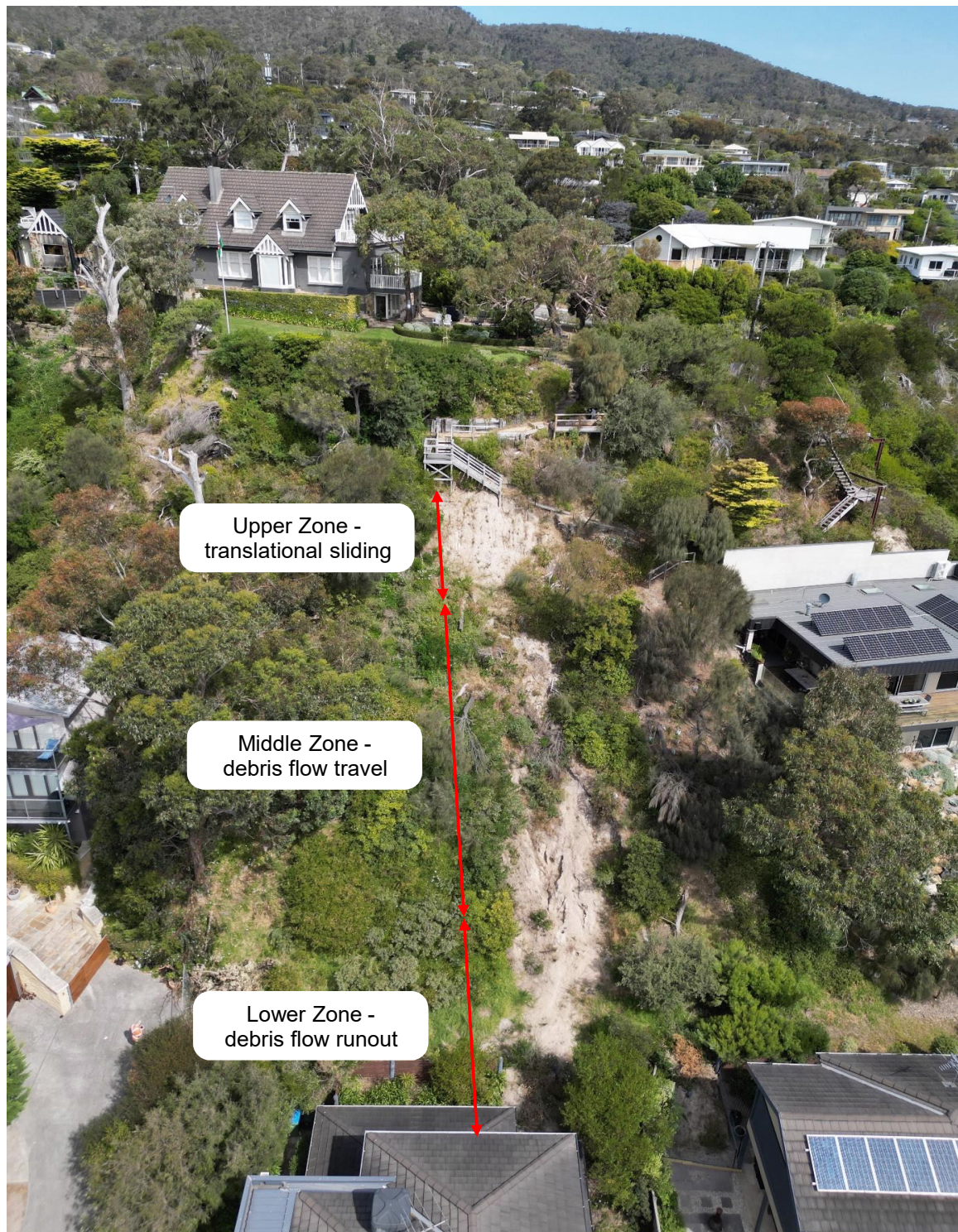
Photo 1 - Landslide Overview, with zones indicated
