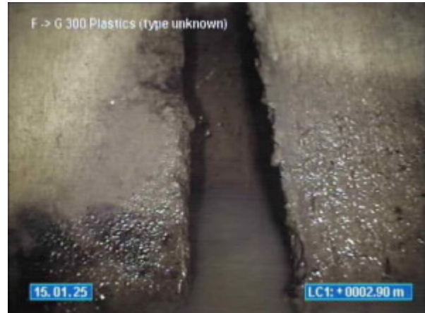
10-12 VIEW POINT ROAD MCCRAE_15.01.2025_142844_F TOO G _055.jpg, 00:01:41, 2.90 Soil visible through defect, at joint
