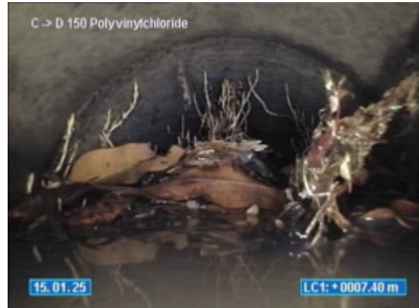
10-12 VIEW POINT ROAD MCCRAE_15.01.2025_104134_C TOO D_019.jpg, 00:07:08, 7.40 Inspection (survey) abandoned, roots
