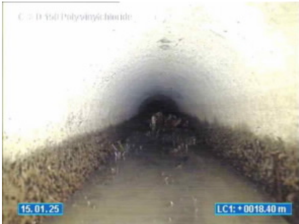
10-12 VIEW POINT ROAD MCCRAE_15.01.2025_114611_C TOO D_029.jpg, 00:04:25, 18.40 Change of conduit material. New material, Fibre reinforced plastic, at joint
