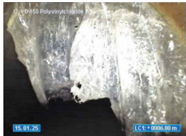
10-12 VIEW POINT ROAD MCCRAE_15.01.2025_114611_C TOO D_024.jpg, 00:04:25, 6.00 Obstruction, an object is intruding through the wall, Obstruction: 80% from 11 o'clock to 4 o'clock
