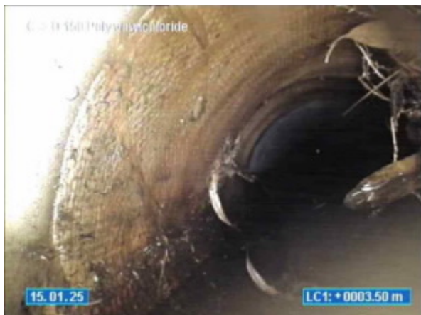
10-12 VIEW POINT ROAD MCCRAE_15.01.2025_104134_C TOO D_017.jpg, 00:02:45, 3.50 Change of conduit material. New material, Fibre reinforced plastic
