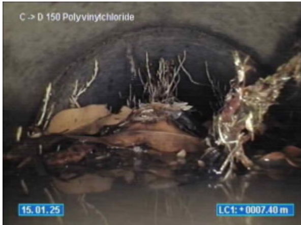
10-12 VIEW POINT ROAD MCCRAE_15.01.2025_104134_C TOO D_020.jpg, 00:05:13, 7.10 Tap roots, reduction in cross sectional area, Obstruction: 50% from 9 o'clock to 3 o'clock
