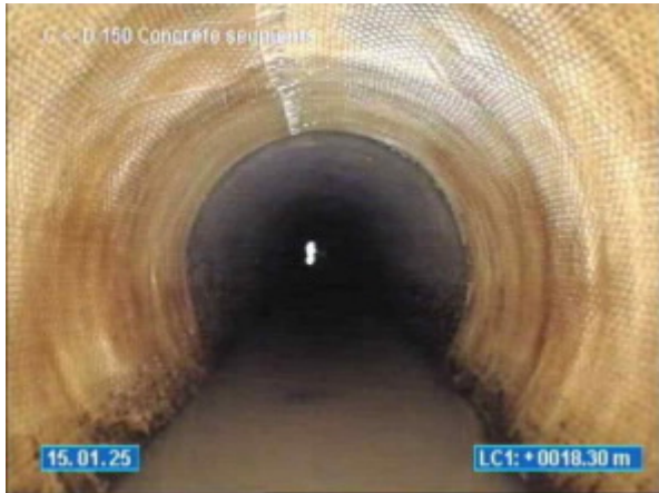
10-12 VIEW POINT ROAD MCCRAE_15.01.2025_132020_D TOO C _041.jpg, 00:33:07, 18.30 Change of conduit material. New material, Fibre reinforced plastic, at joint
