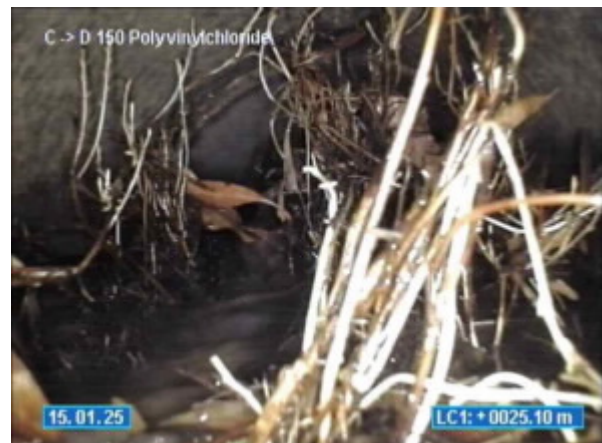
10-12 VIEW POINT ROAD MCCRAE_15.01.2025_114611_C TOO D_032.jpg, 00:00:00, 25.10 Inspection (survey) abandoned, roots
