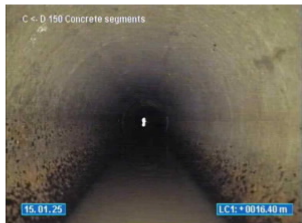
10-12 VIEW POINT ROAD MCCRAE_15.01.2025_132020_D TOO C _040.jpg, 00:33:07, 16.40 Change of conduit material. New material, Concrete reinforced, at joint
