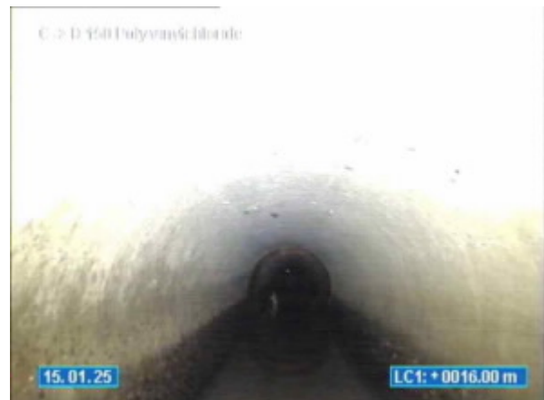
10-12 VIEW POINT ROAD MCCRAE_15.01.2025_114611_C TOO D_028.jpg, 00:04:25, 16.00 Change of conduit material. New material, Concrete segments, at joint
