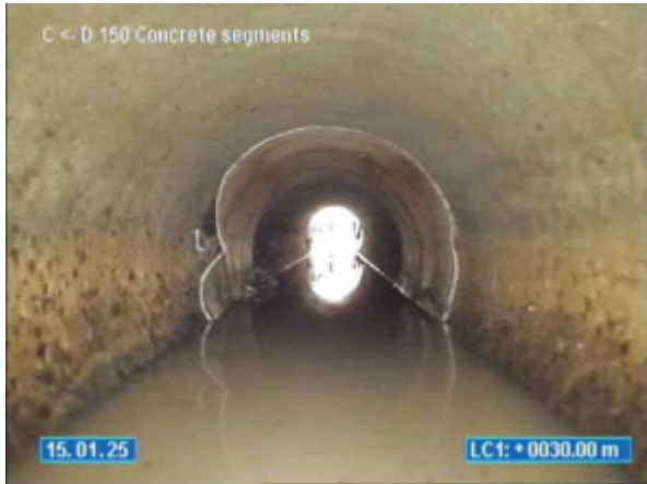
10-12 VIEW POINT ROAD MCCRAE_15.01.2025_132020_D TOO C _045.jpg, 00:33:07, 30.00 Change of conduit material. New material, Concrete reinforced, at joint
