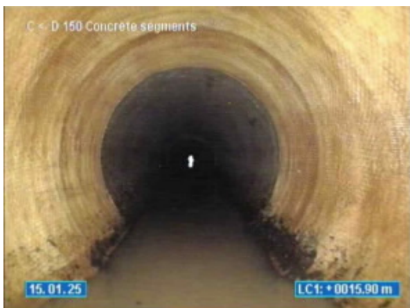
10-12 VIEW POINT ROAD MCCRAE_15.01.2025_132020_D TOO C _039.jpg, 00:33:07, 15.90 Change of conduit material. New material, Fibre reinforced plastic, at joint
