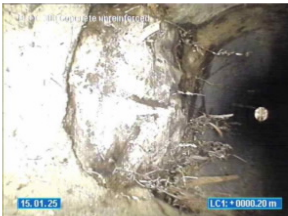
10-12 VIEW POINT ROAD MCCRAE_15.01.2025_102122_B TOO C _010.jpg, 00:02:28, 0.20 Breaking, all pieces are present but some of them are visibly displaced from position, length of break: 300mm from 11 o'clock to 1 o'clock
