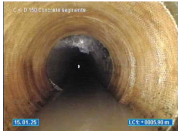
10-12 VIEW POINT ROAD MCCRAE_15.01.2025_132020_D TOO C _038.jpg, 00:33:07, 5.90 Change of conduit material. New material, Fibre reinforced plastic, at joint
