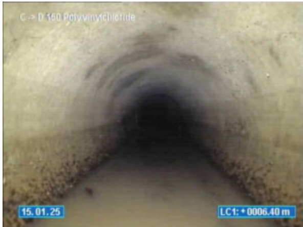
10-12 VIEW POINT ROAD MCCRAE_15.01.2025_114611_C TOO D_025.jpg, 00:04:25, 6.40 Change of conduit material. New material, Concrete segments, at joint
