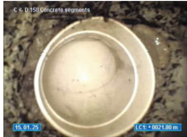
10-12 VIEW POINT ROAD MCCRAE_15.01.2025_132020_D TOO C _042.jpg, 00:33:07, 21.80 Connection, unlined, connection appears to be open, Height/Diameter (mm): 150 at 12 o'clock
