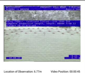
Observation Code: RPL Point repair, localised lining--less than the complete inspection length, length: 600mm from 12 o'clock to 12 o'clock
