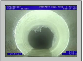
Location of Observation: 7.03m Video Position: 00:00:49 Observation Code: RPL[PHOTO 2] Point repair, localised lining--less than the complete inspection length, length: 600mm from 12 o'clock to 12 o'clock
