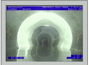
Location of Observation: 29.07m Video Position: 00:03:35 Observation Code: RPL[PHOTO 2] Point repair, localised lining--less than the complete inspection length, length: 600mm from 12 o'clock to 12 o'clock
