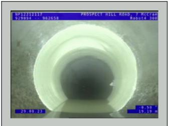
Location of Observation: 19.19m Video Position: 00:02:36 Observation Code: RPL[PHOTO 2] Point repair, localised lining--less than the complete inspection length, length: 600mm from 12 o'clock to 12 o'clock
