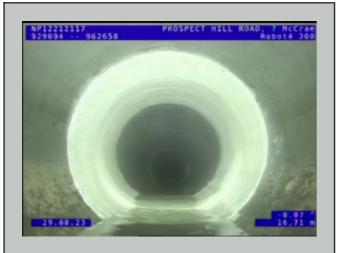
Location of Observation: 16.71m Video Position: 00:02:05 Observation Code: RPL[PHOTO 2] Point repair, localised lining--less than the complete inspection length, length: 600mm from 12 o'clock to 12 o'clock
