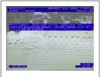
Location of Observation: 19.14m Video Position: 00:03:09 Observation Code: RPL Point repair, localised lining--less than the complete inspection length, length: 600mm from 12 o'clock to 12 o'clock
