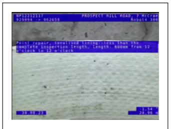
Location of Observation: 28.96m Video Position: 00:04:07 Observation Code: RPL Point repair, localised lining--less than the complete inspection length, length: 600mm from 12 o'clock to 12 o'clock
