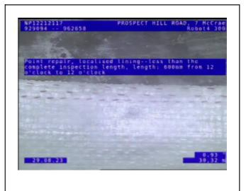
Location of Observation: 30.32m Video Position: 00:04:00 Observation Code: RPL Point repair, localised lining--less than the complete inspection length, length: 600mm from 12 o'clock to 12
