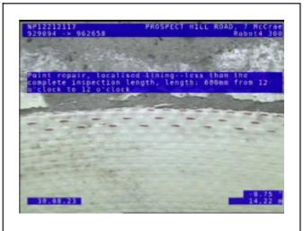
Location of Observation: 14.22m Video Position: 00:01:47 Observation Code: RPL Point repair, localised lining--less than the complete inspection length, length: 600mm from 12 o'clock to 12 o'clock
