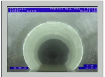
Location of Observation: 14.33m Video Position: 00:01:34 Observation Code: RPL[PHOTO 2] Point repair, localised lining--less than the complete inspection length, length: 600mm from 12 o'clock to 12 o'clock
