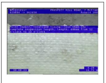
Location of Observation: 16.71m Video Position: 00:02:33 Observation Code: RPL Point repair, localised lining--less than the complete inspection length, length: 600mm from 12 o'clock to 12 o'clock
