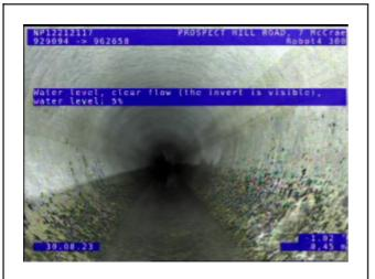
Location of Observation: 0.45m Video Position: 00:00:17 Observation Code: WLC Water level, clear flow (the invert is visible), water level: 5%
