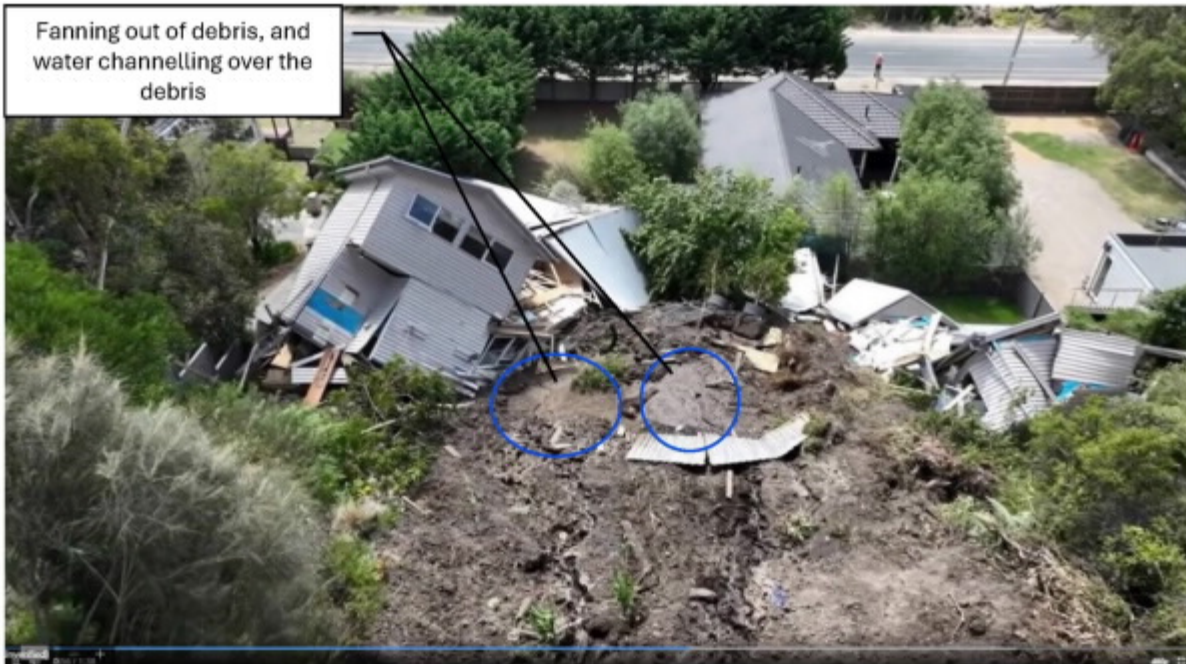
Figure 18: Drone footage, showing the toe debris.
