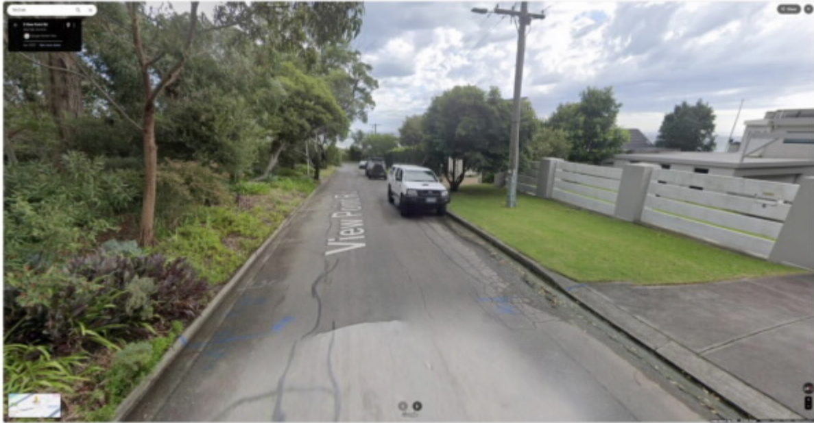
Figure 6: Google Streetview image from April 2023 looking west from outside No. 6 View Point Road. Note the localised spalling and crocodile cracking of the pavement adjacent to the driveway of No. 6.
