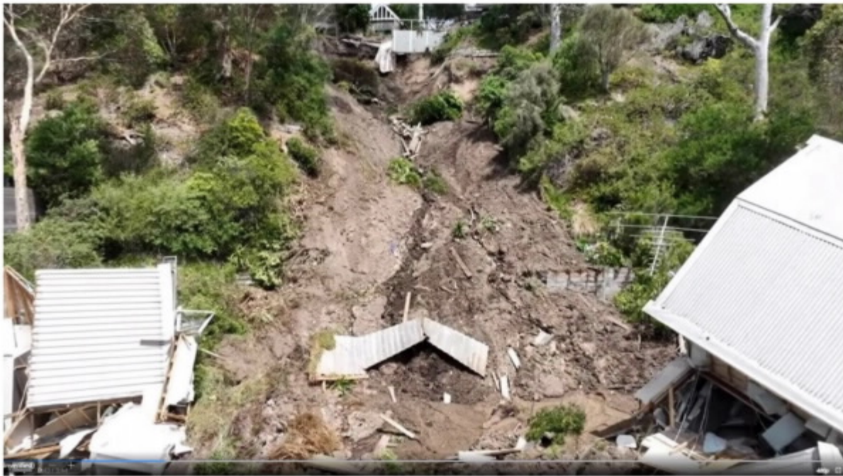
Figure 11: Drone footage taken from toe of failure, illustrating the 'bowl' shaped failure within the upper slope.
