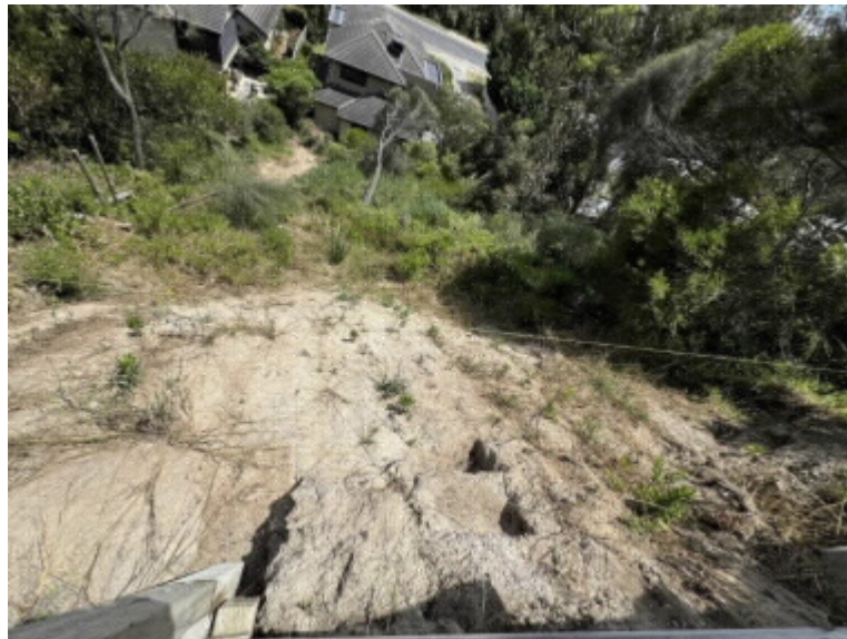
Figure 9: Dried out head scarp (photograph taken 4 December 2023)
